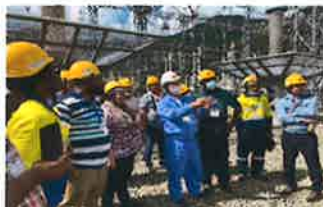
At 500kV substation
