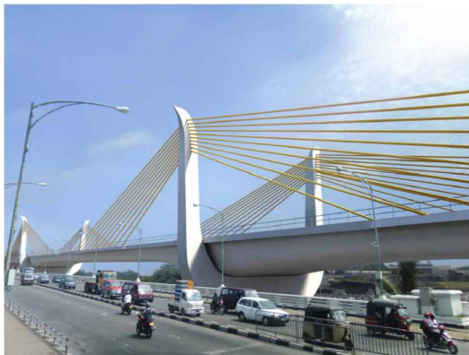
Main Bridge (Extradosed)
