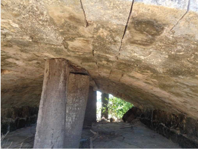
Arch propped by timber logs
