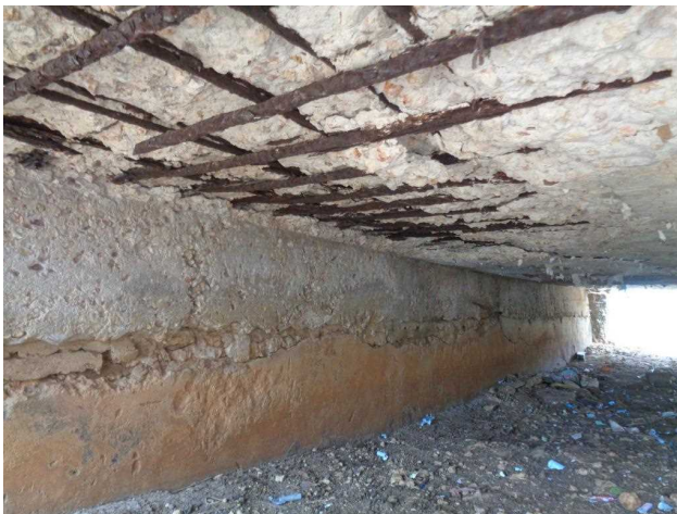
Reinforcement exposed
