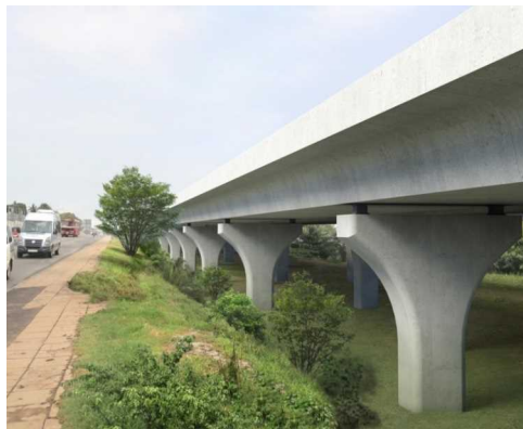
Approach Bridge (PC Box Girder)
