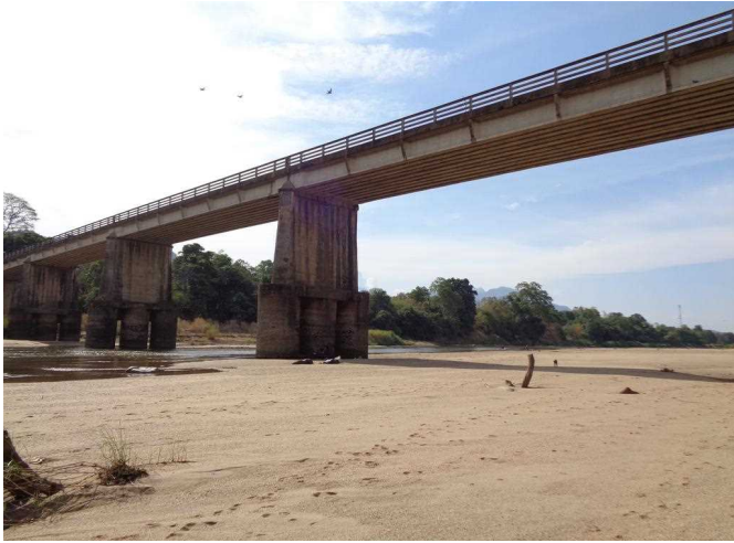
General view of the bridge
