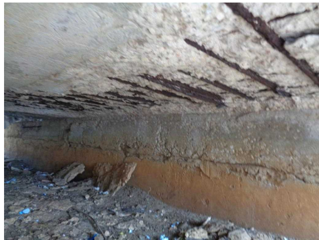
Reinforcement exposed
