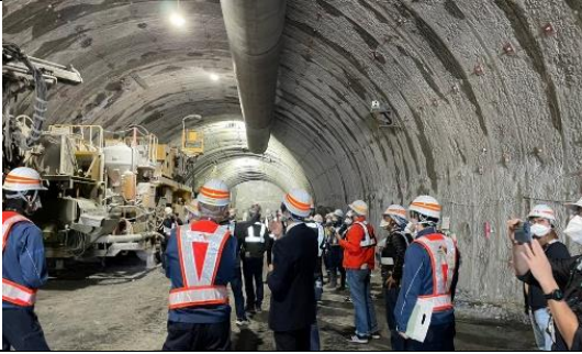
21 November NEXCO Central Yoro Tunnel Observation 1
