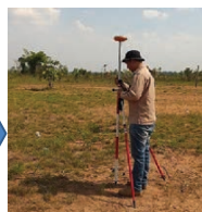
Geo Base (GNSS) setting on a benchmark
