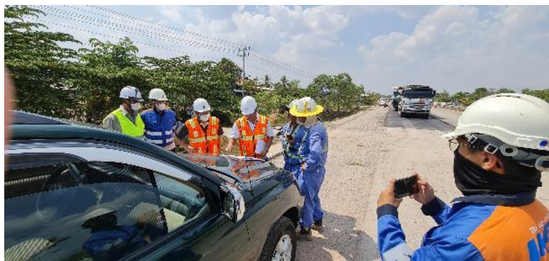
Figure 2-6 Meeting for surveying plan with Construction surveying team
