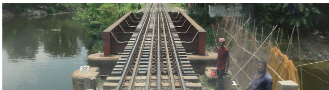
Figure 6.11 Steel Plate / Steel Semi-Through Plate Girders with Brick Piers / Abutments (Bridge No.33)
