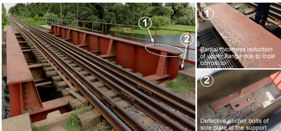
Figure 6.16 Thickness Reduction due to Corrosion / Defective Anchor Bolts (Bridge No.35)
