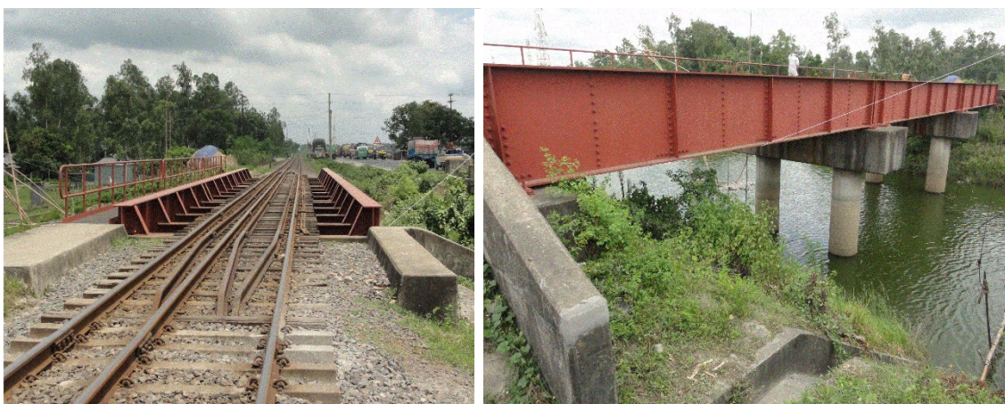
Figure 6.6 Steel Semi-Through Plate Girders with RC Piers / Abutments (Bridge No.119)
