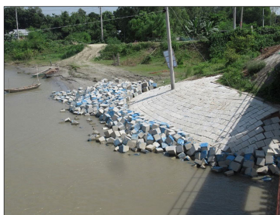
River Training Work (under construction)
