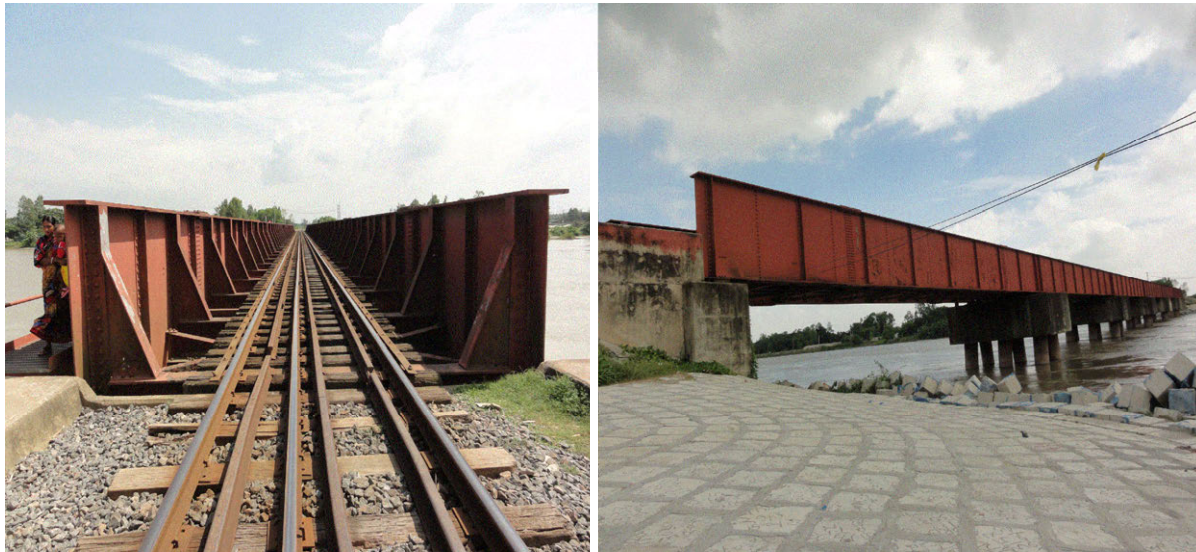
Figure 6.7 Steel Semi-Through Plate Girders with RC Piers / Abutments (Bridge No.98)
