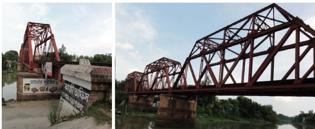
Figure 6.14 Steel Plate / Steel Through Truss Girders with Brick Piers / Abutments (Bridge No.23)
