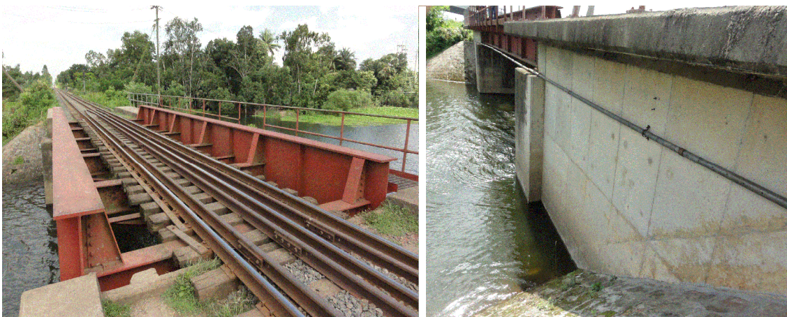
Figure 6.5 Steel Semi-Through Plate Girder with RC Abutments (Bridge No.35)
