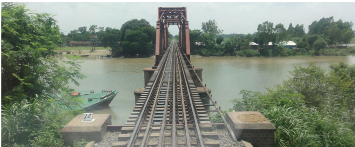
Figure 6.13 Steel Plate / Steel Through Truss Girders with Brick Piers / Abutments(Bridge No.24)
