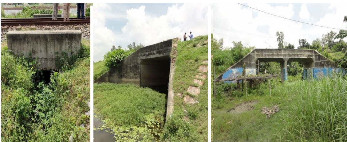
Figure 6.15 RC Box Culverts (Bridge No.119/20, 41A, 120 from the left)
