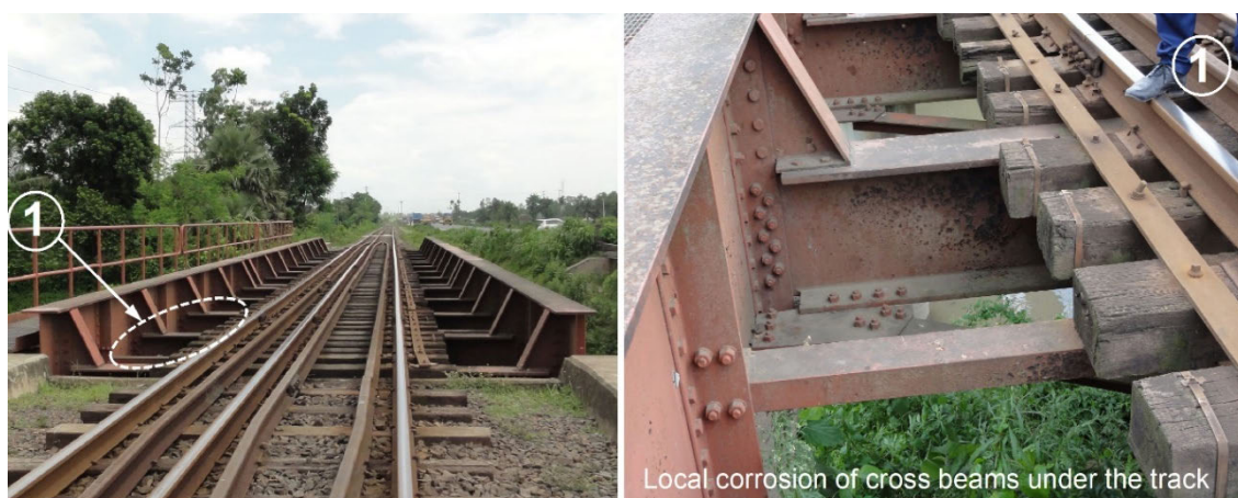
Figure 6.17 Local Corrosion due to Organic Excrement from Passing Trains (Bridge No.116)
