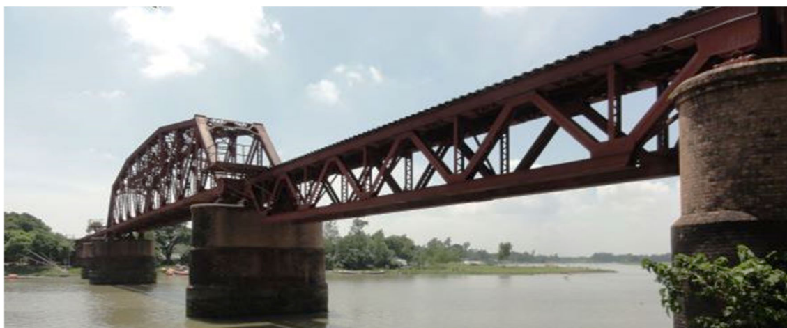
Figure 6.11 Steel Plate / Steel Semi-Through Plate Girders with Brick Piers / Abutments (Bridge No.33)
