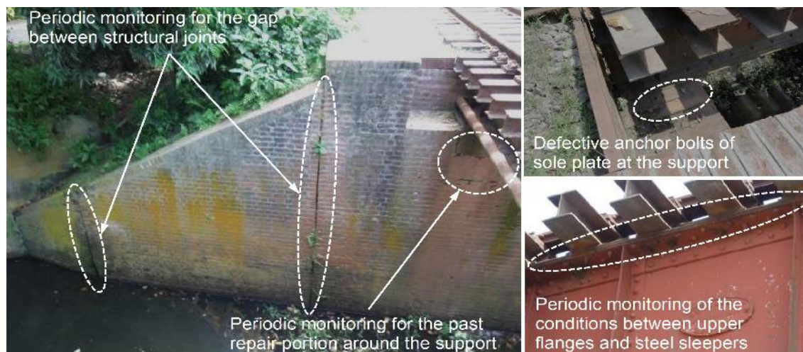
Figure 6.19 Periodic Monitoring Items Required / Defective Anchor Bolts (Bridge No.34 constructed in 1914)
