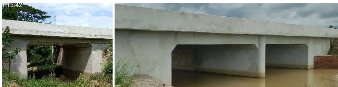
Figure 6.21 Examples of Construction of New Box Culverts
