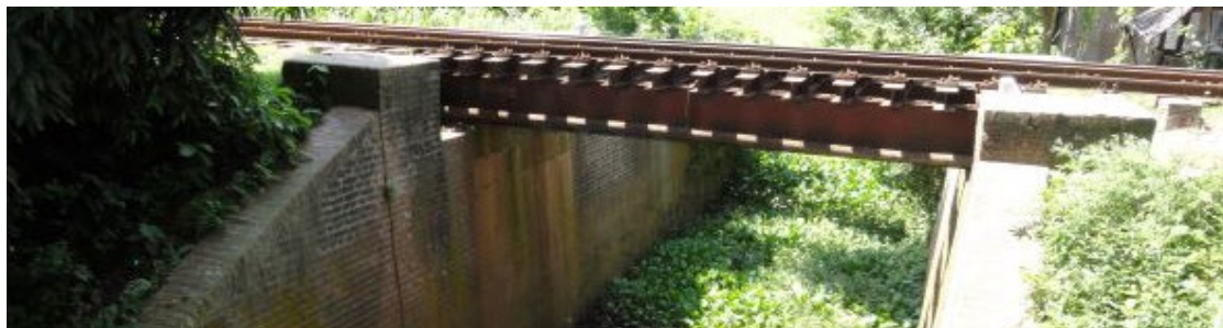
Figure 6.9 Steel Plate Girder with Brick Abutments (Bridge No.34)
