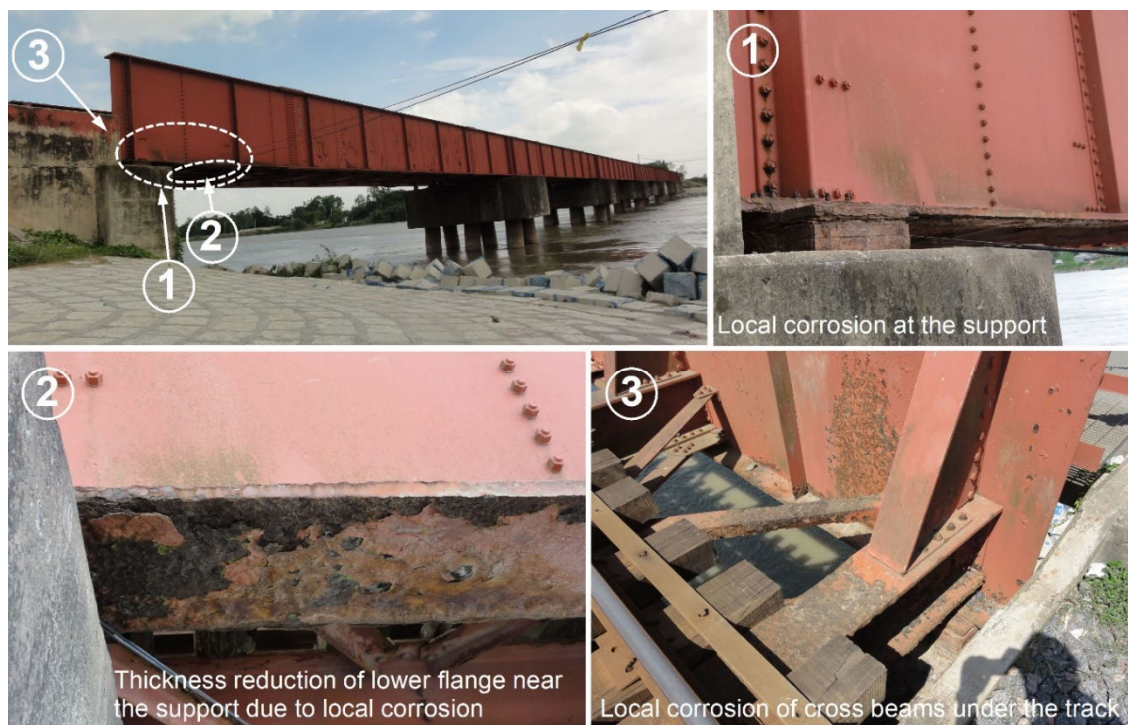
Figure 6.18 Local Corrosion due to Wet-dry Cyclic and Organic Excrement (Bridge No.98)
