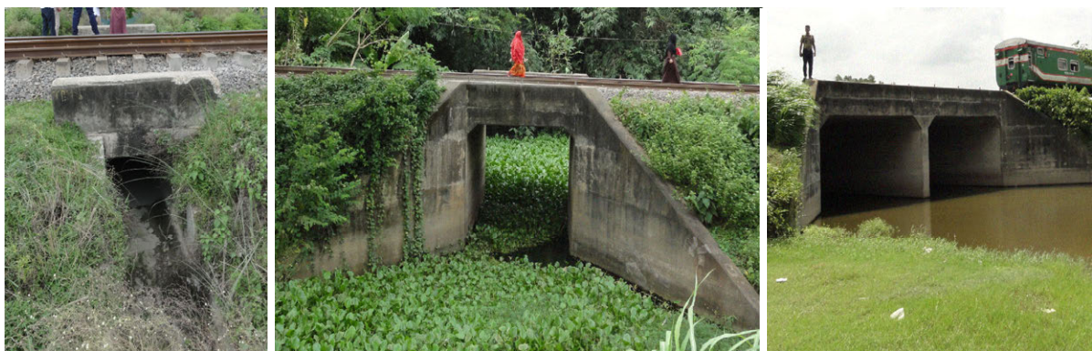
Figure 6.8 RC Box Culverts (Bridge No.119/2, 48, 114 from the left)
