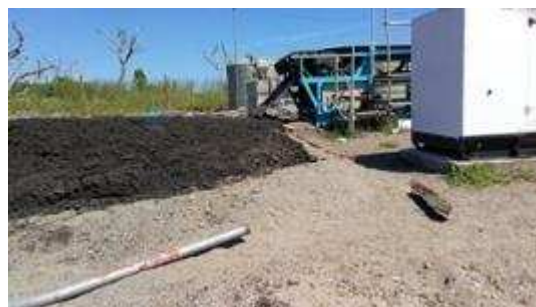
Drying Sludge Dredged from the Stabilization Pond
