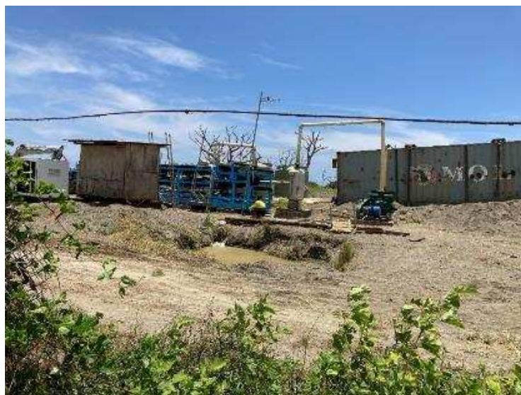
Photo 4-3.1 Dewatering of Dredged Sludge at Olosara WWTP
