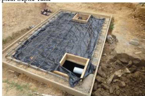
Construction of Septic Tank
