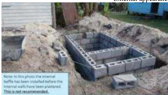
Construction of Septic Tank
