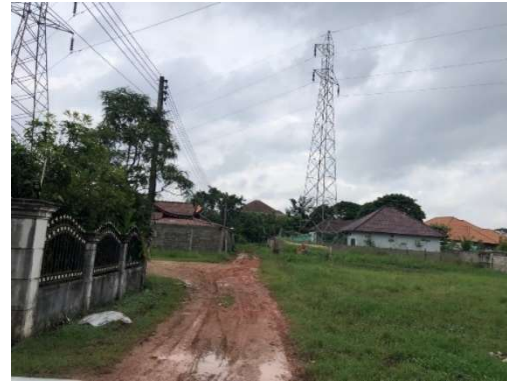
High Voltage Transmission Line
