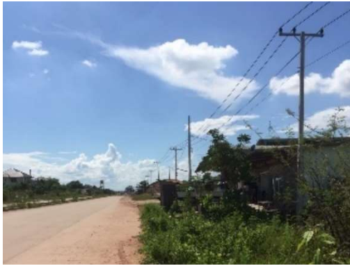
22 KV Electric Line
