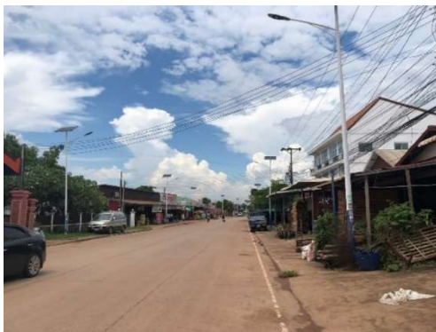
Concrete Paved Road (Outer Trunk Road)
