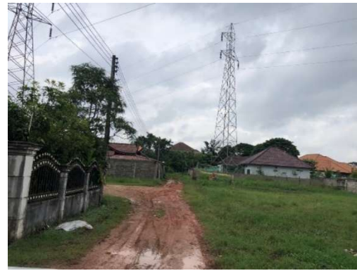
High Voltage Transmission Line
