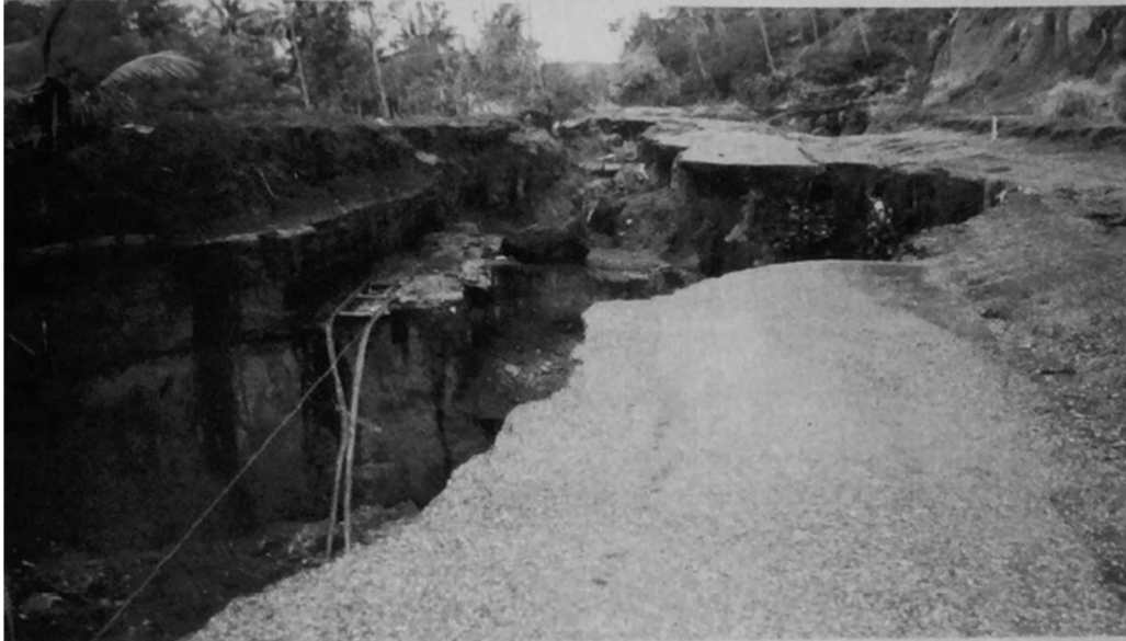
Figure 5.3.5 Effect of Mudflow Along Namanula Road in Rabaul During 1994 Eruption
