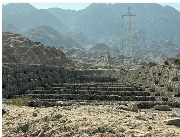
Figure 6-22 Wadi that was creating as a flash flood protection in the urban fringe area
