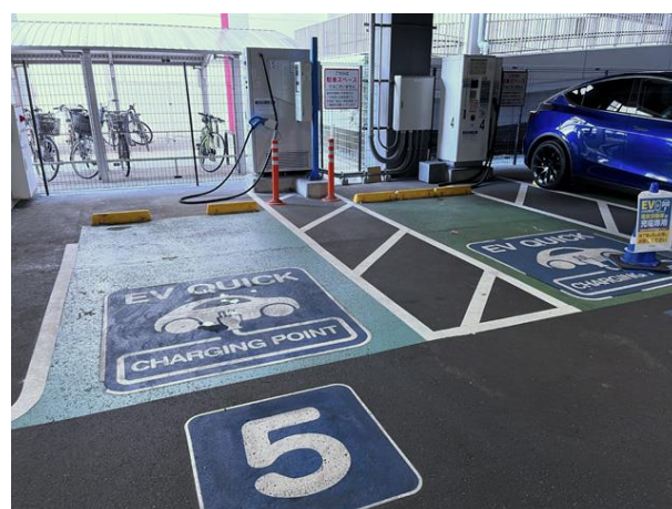
Figure 7-58 EV Quick Charging Devices in a Commercial Building (Japan)
