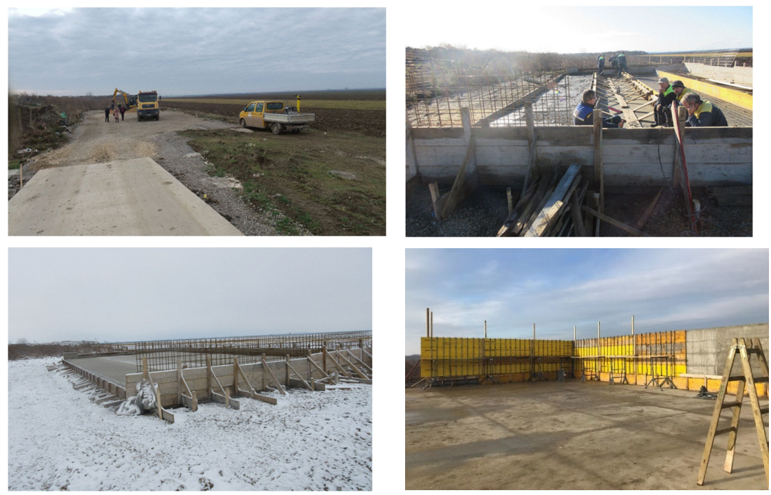
Figure 79 RY under Construction
