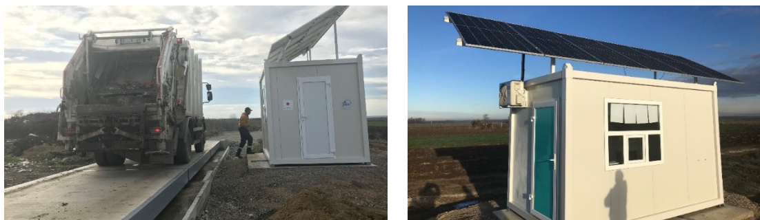
Figure 80 Constructed Weighbridge and its Control House
