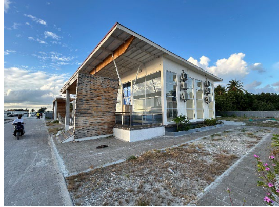
Terminal building (Side View)
