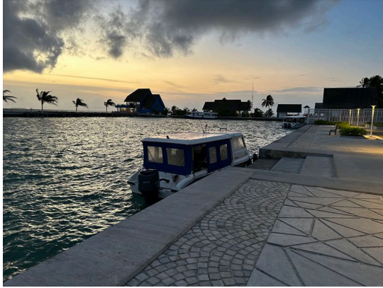
Mooring Facilities (Revetment with Steps)
