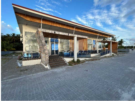
Terminal Building (Front)
