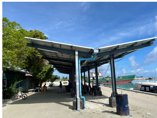
Freight Handling Facility with Solar Power Generation
