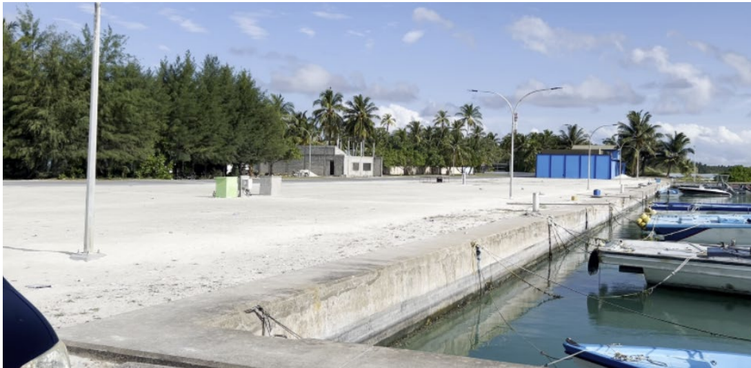
Mooring Facility, Gas station
