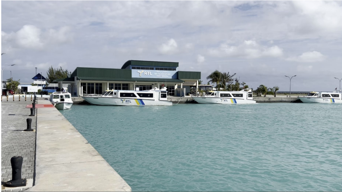
Panoramic View of Kulhudhuffushi (hub terminal)
