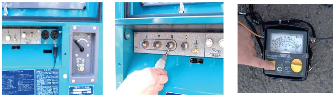
Connect clip to body ground/ Connect plug to output terminal/ Push measure button, and measure
