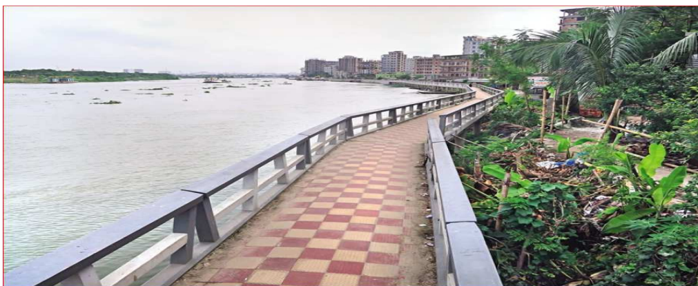
Photo 33: Newly Built Walkway by BIWTA
