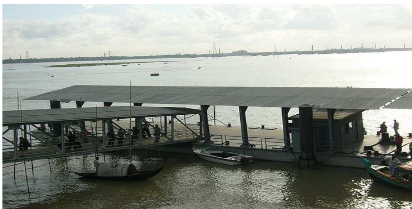
Photo 29: Ashulia Landing station During Monsoon, Dhaka
