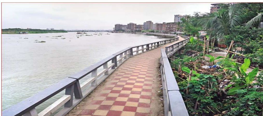
Photo 3: Riverside walkway works in Progress by BIWTA
