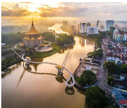
Photo 22: The Darul Hana Bridge spanning the north and south bank (Kuching Waterfront) of the Sarawak river
