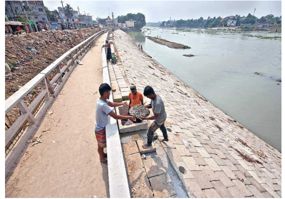
Photo 35: Walkway Construction in Progress (River Turag) (BIWTA)
