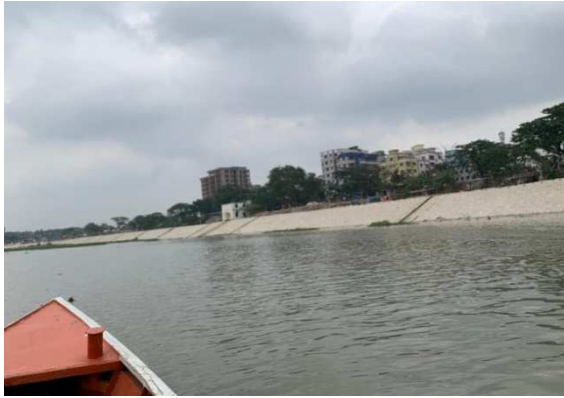
Photo 34: River Protection Project work in progress (River Turag) (BIWTA)
