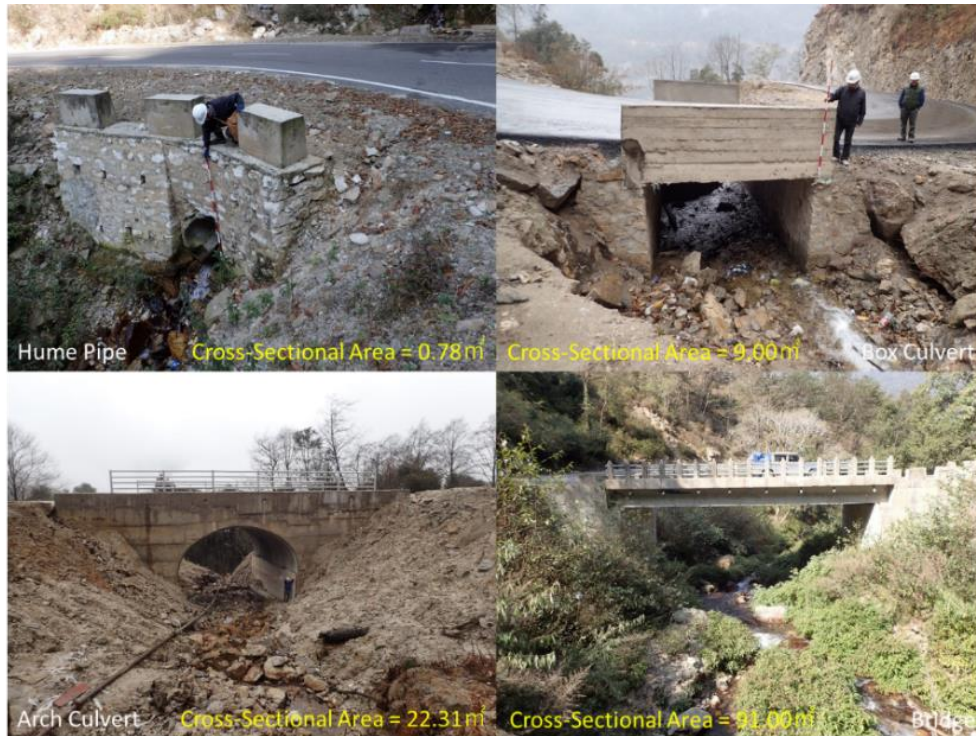
*1 Upper left: Hume pipe *2 Upper right: Box culvert *3 Lower left: Arch culvert *4 Lower right: Bridge (Source: JET)
