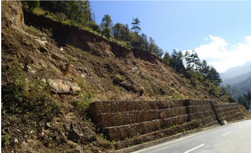
(Source: JET) Photo 3.5-3 Reinforced Soil Wall Falling Rock Protection Wall Completed (2020/11/5)
