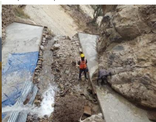
Placement of concrete for abut foundation (Apr/12/2020)
