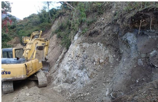
Construction of access roads
