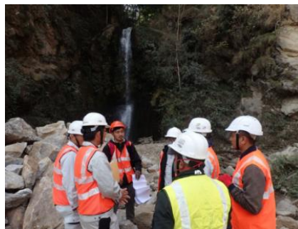
On-site meeting before construction (Feb/13/2020)
