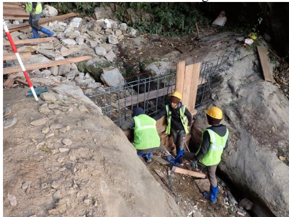
Construction of intake weir (Jan/13-20/2023)
