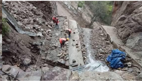
Start masonry work on left bank abutment(Apr/26/2020)
