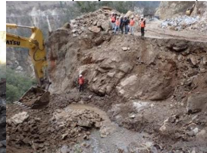
Excavation of culvert installation area completed (Mar/8/2020)
