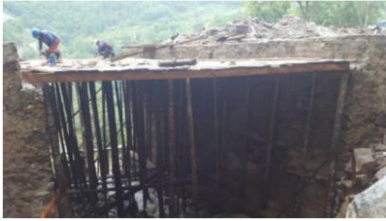
Installation of Slab Shoring (Jun/29/2020)
