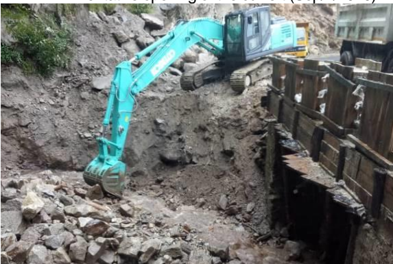
Start of left-bank wing wall construction (Sep/26/2020) (Source: JET)
