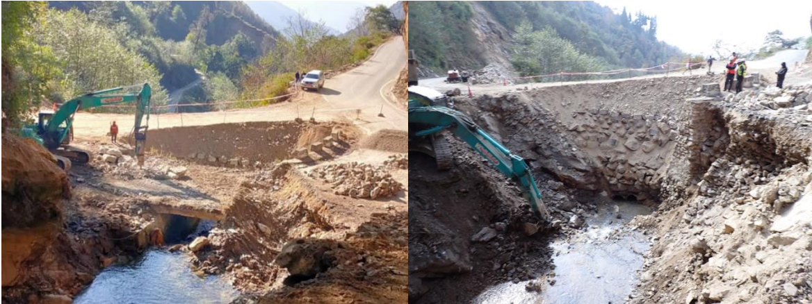
Start of removal of existing culvert (Jan/2/2023)
