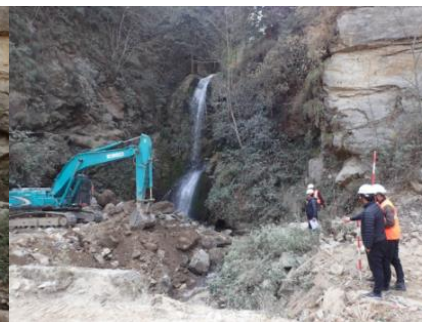
Start of temporary road construction (Feb/18/2020)
