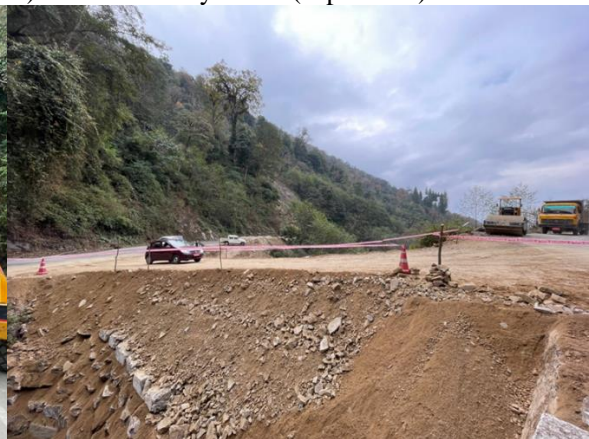
Opening of bypass (Dec/31/2022)
