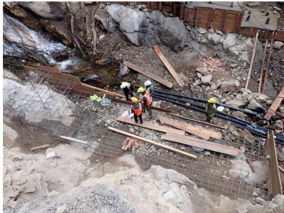
Construction of right bank abut foundation section (Jan/16-Feb/7/2023)
