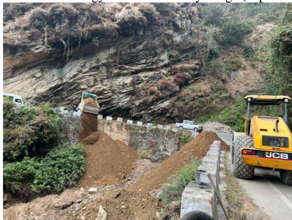
Start construction of bypass (Dec/24/2022)
