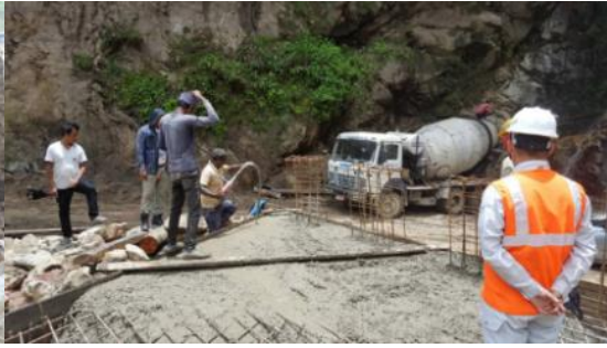
Slab Concrete Placement (Jul/15/2020)
