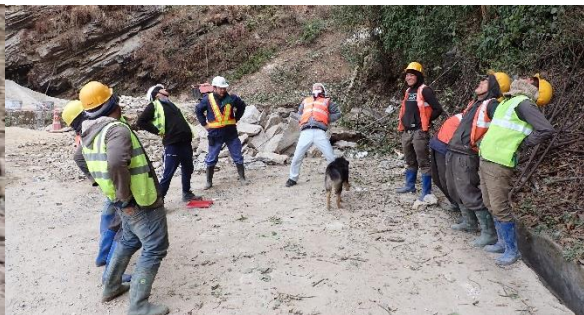
Preparatory exercises before works
