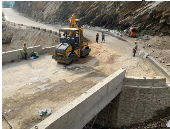
Roadbed grading and paving (Apr/23-May/4/2023)
