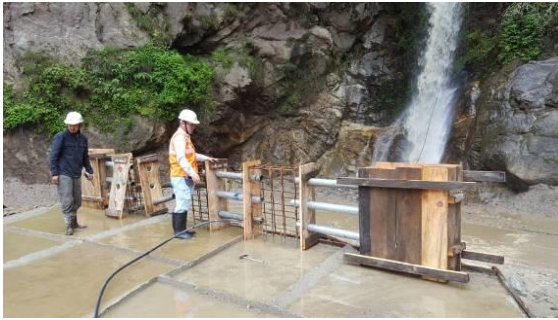
Construction of Parapet (Jul/18/2020)
