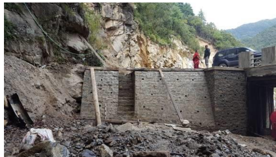
Completion of left-bank wing wall construction (Oct/24/2020)
