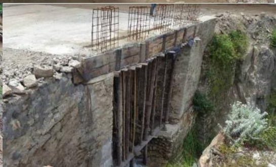
Panoramic view of the culvert (Sep/8/2020)
