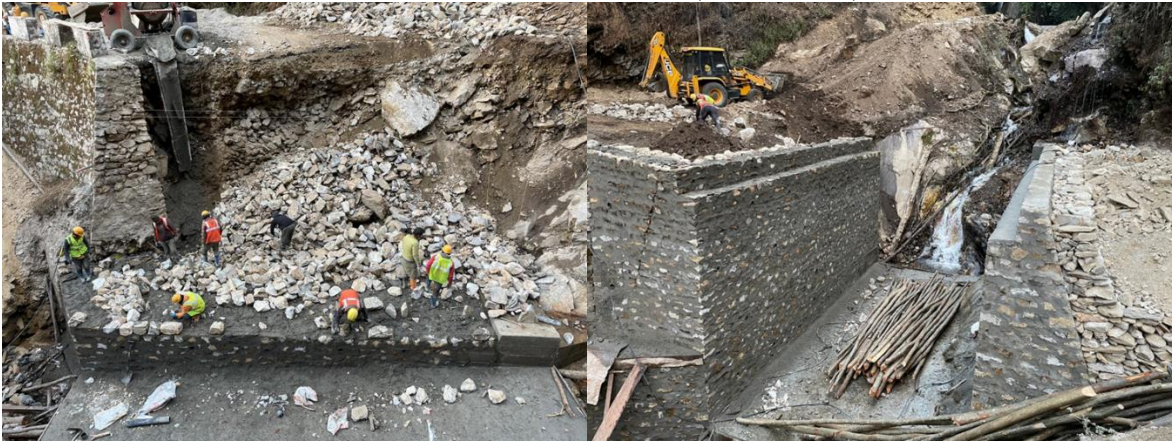
Construction of right bank abutments (Feb/15-23/2023)
