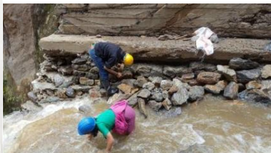
Emergency restoration work for damaged areas (Jun/19/2020)
