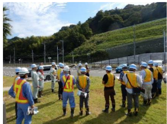
By West Nippon Expressway Engineering Chugoku Co. Explanation of the site where the debris flow occurred (9/25/2019)
