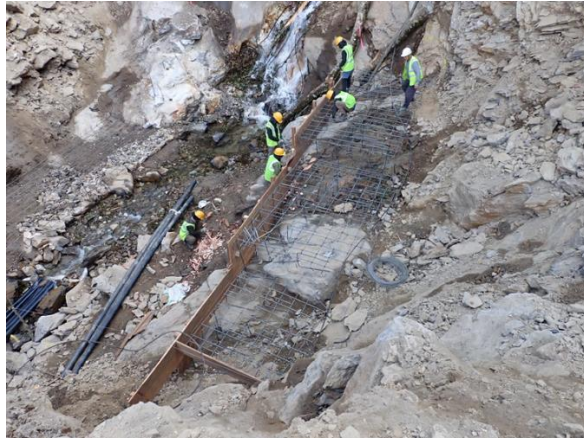
Construction of left bank abut foundation section (Jan/16-Feb/7/2023)
