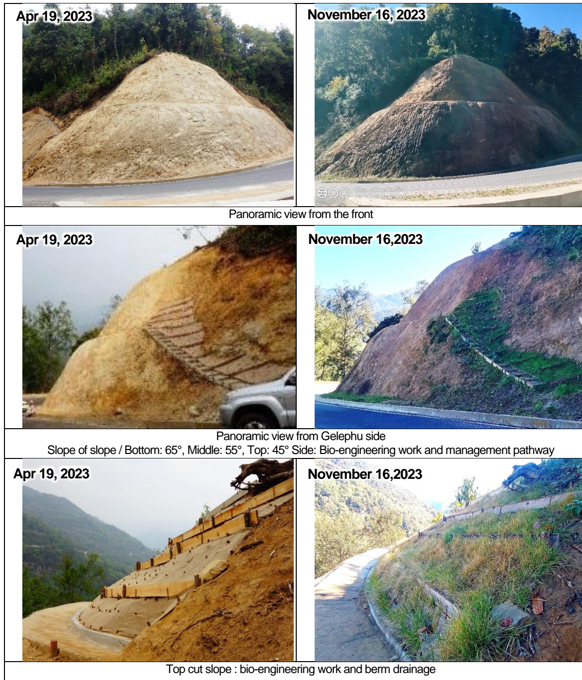
Photo 3.4-16 Cut slope construction on output 3 / post-completion and current conditions
