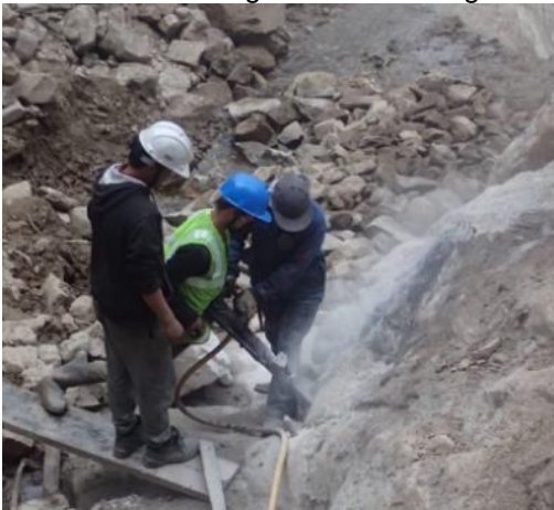
Anchor hole installation status at right bank foundation (Mar/17/2020)
