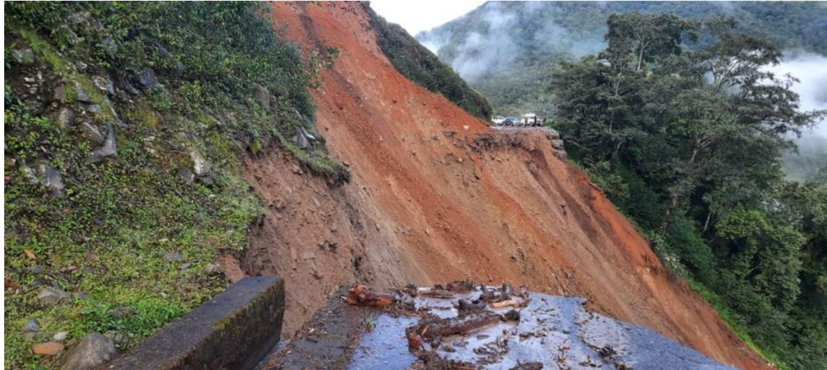
Huge landslide in Khelekha area caused by debris flow that washed down the road surface (Sep/15/2021)
