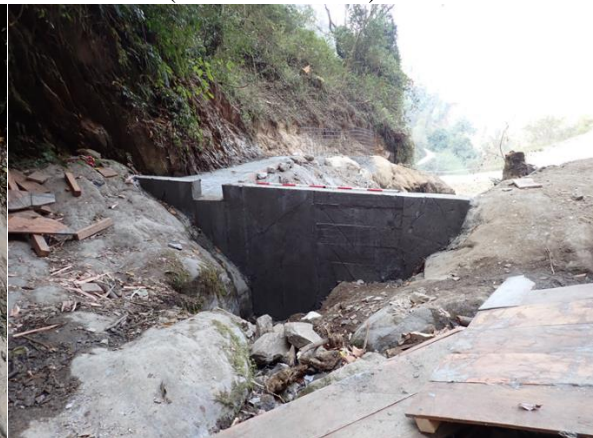
Construction of intake weir (Jan/13-20/2023)
