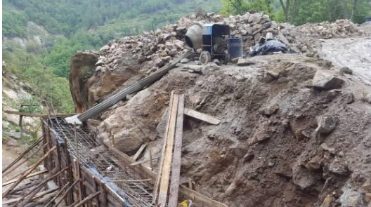
Concrete Poured for Right Bank Abutments (May/23/2020)
