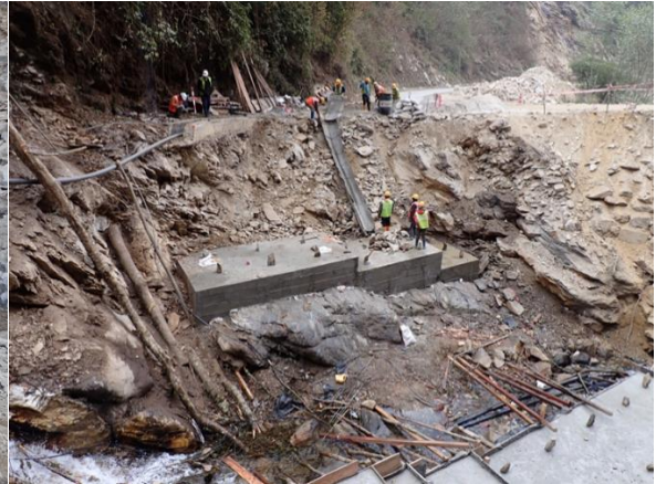
Construction of left bank abut foundation section (Jan/16-Feb/7/2023)
