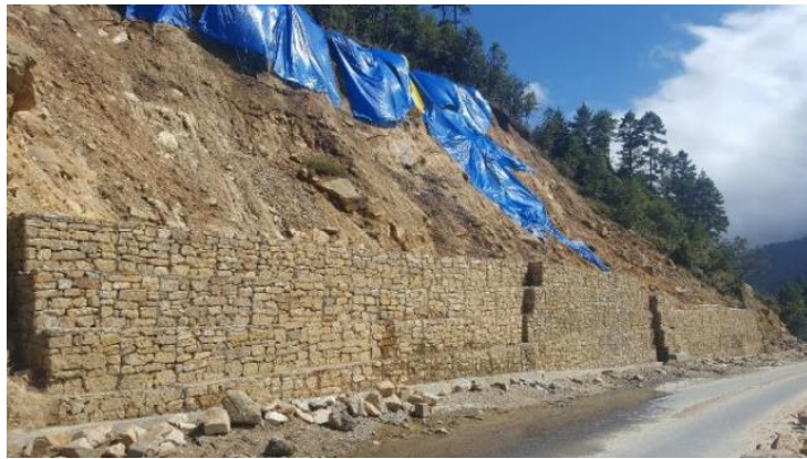
Photo 3.5-7 Slope protection with blue sheets (10/8/2020)
