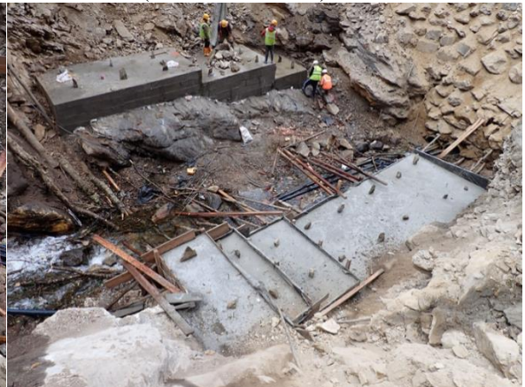
Construction of right bank abut foundation section (Jan/16-Feb/7/2023)
