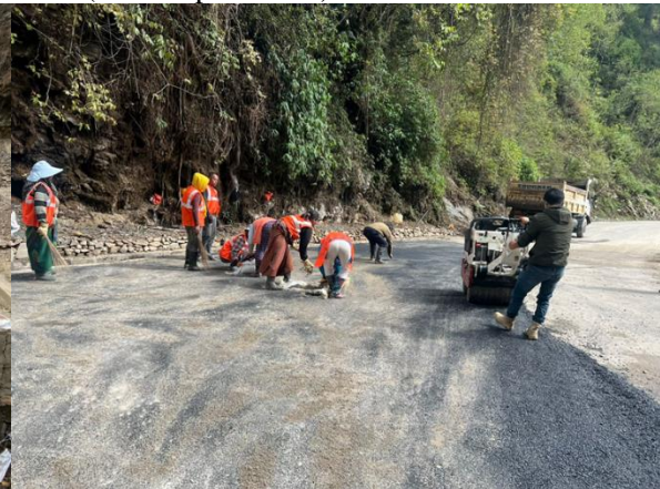
Roadbed grading and paving (Apr/23-May/4/2023)
