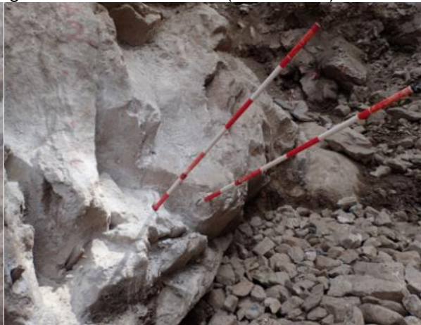
Anchor hole installation status at right bank foundation (Mar/17/2020)
