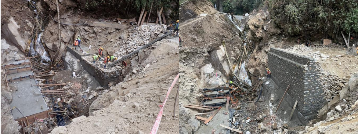
Construction of left bank abutments (Feb/8-12/2023)
