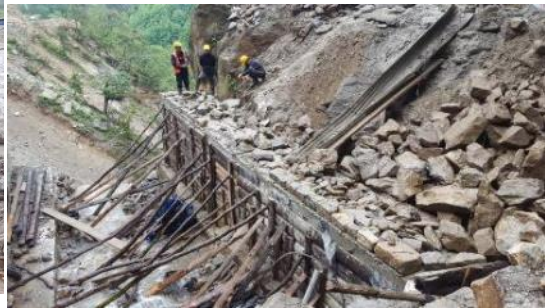
Masonry work on the Right Bank Abutment Begins (May/26/2020)
