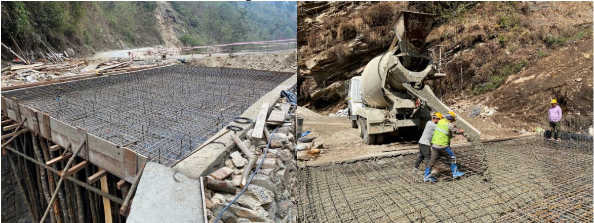
Slab shoring and slab construction (Feb/24-Mar/3/2023)
