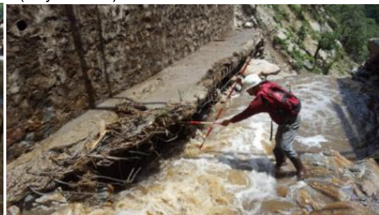
Culvert abutments completed on left and right bank (Jun/12/2020)
