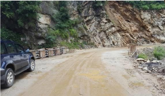
Tentative opening of the culvert (Sep/7/2020)
