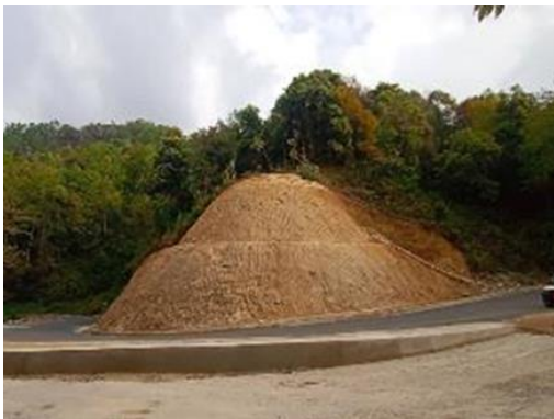
Output 3: Completion of cut-and-fill construction site (Apr 27, 2023)
