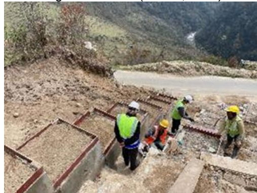
Result 2: Construction status of drainage works (Mar 25, 2023)
