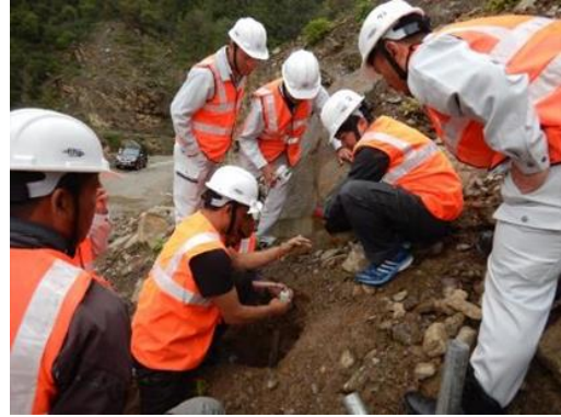
Output 1: Technical transfer seminar on installation of inclinometer (Apr 26, 2019)
