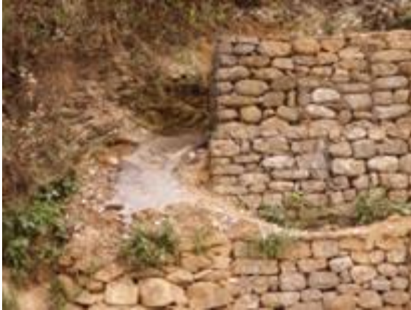
Figure3.3-67 Cascade drain (CD6) 0.5~1.0 (W)x1.50 (L) >0.47m (W)x 1.84m(L).
