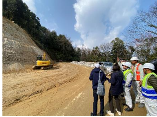
Output 3: JICA headquarters construction site visit (Mar 6, 2023)
