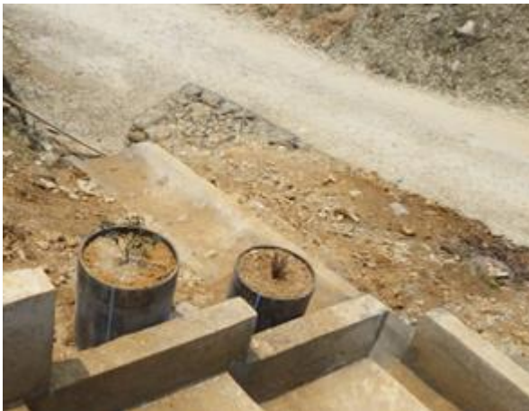
Figure3.3-67 Cascade drain (CD6) 0.5~1.0 (W)x1.50 (L) >0.47m (W)x 1.84m(L).
