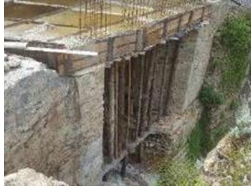
Result 5: Construction for countermeasures against debris flows (Aug 5, 2020)
