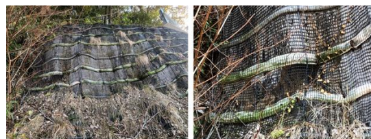
Photo 3.3-12 Rock Revegetation Work on Steep Slope (Hasuike, Tosa City). 33°29'7.75"n, 133°24'20.11"e
