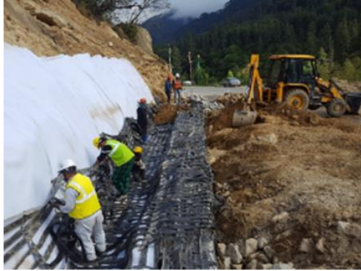
Result 4: Construction of rockfall prevention work (May 7, 2020)
