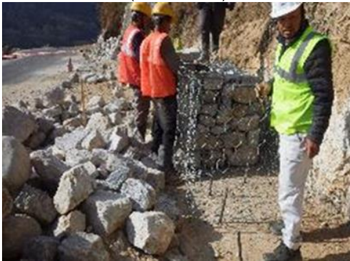
Result 2: Start of the second test construction (Jan 25, 2023)
