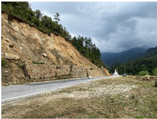
Output 4: Completion of rockfall prevention work (May 8, 2020)
