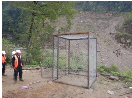
Setting up the protective fence
