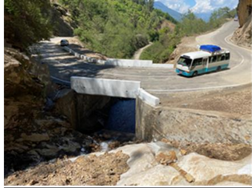
Output 5: Completion of culvert construction (May 5, 2023)
