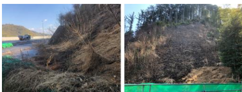
Photo 3.3-11 Rock greening work (East of Tenjin IC, Kochi Expressway). 33°32'34.99"N, 133°25'55.9"E
