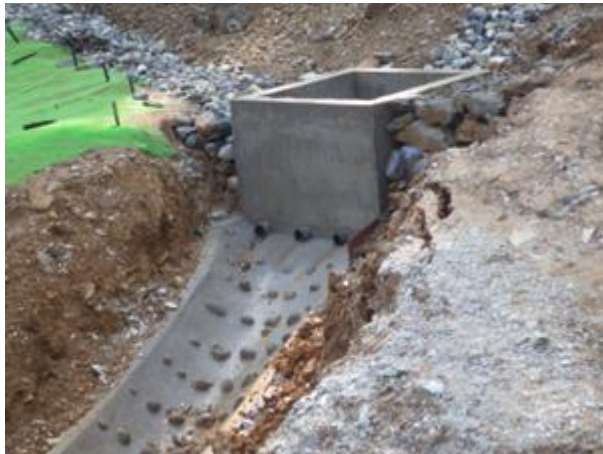
Figure3.3-72 Energy reducer (ER1) Box type , 1,500x1,500, \succ 1,520 \times 1,500 , Thickness: 15~16cm.
