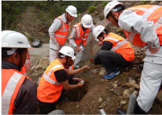
Install the tilt sensor
