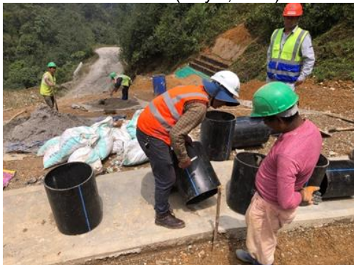
Result 2: Status of the third test construction (Apr 1, 2024)
