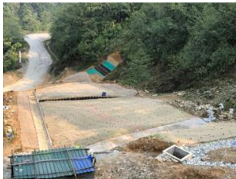
Photo 3.3-44 Berm drain from construction site information (Br 1 and Br 2 are visible).
