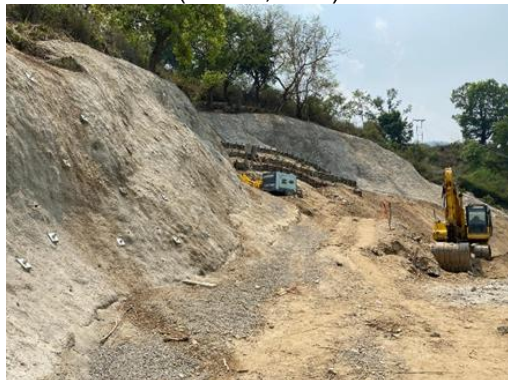
Output 4: Completion of spraying work (Apr 28, 2024)
