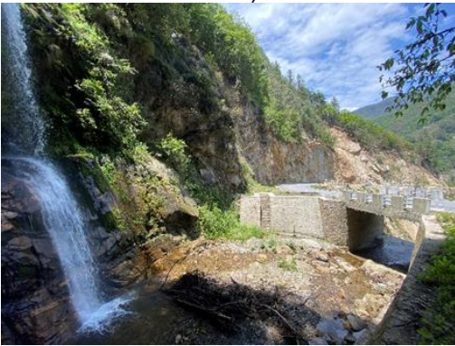
Output 5: Completion of culvert construction (May 8, 2020)
