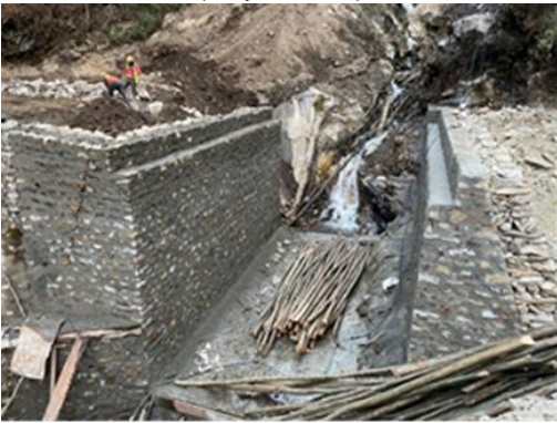
Result 5: Construction of left and right bank abutments (Feb 23, 2023)
