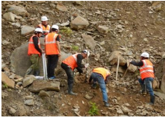
Digging to install the tilt sensor
