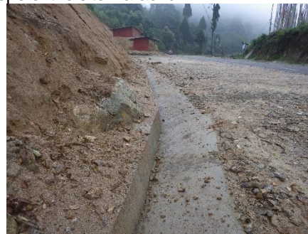
Photo 3.3-5 The drain at the foot of the slope.
