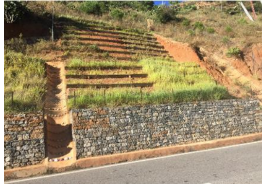
Result 2: Completion of the first test construction of vegetation works (Oct 31, 2020)
