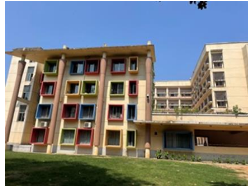
The children's home (girls' dormitory) in Dhaka. The facility has a capacity for 175 children and currently accommodates 130
