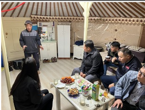
Inside the Ger house Hot water is circulated from the water heater. An electric heater is also installed as a backup.
