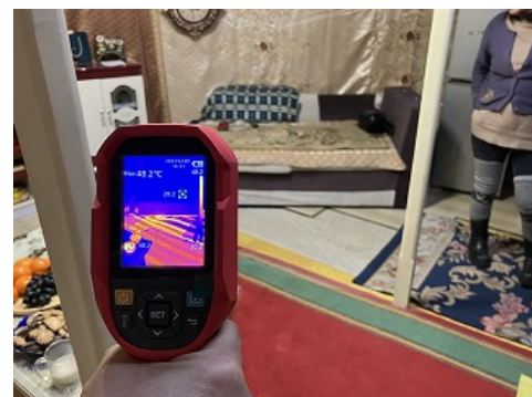
Temperature inside the Ger (December) The floor is very warm due to underfloor heating (red), while the wall is cooler (blue).
