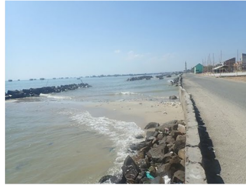
Breakwater Lepas Pantai
