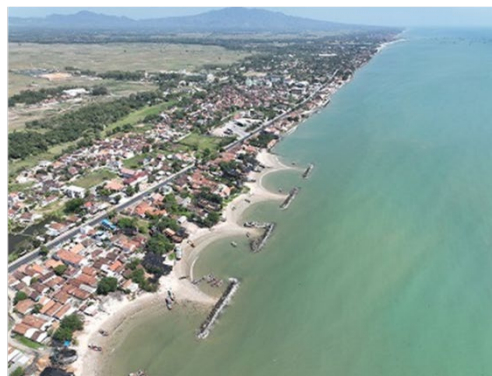
Breakwater Lepas Pantai
