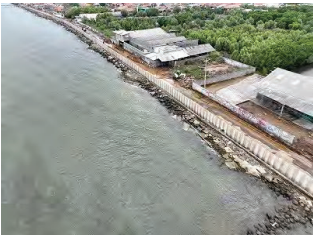
Coastal Protection at Urban Area (Line Protection)
