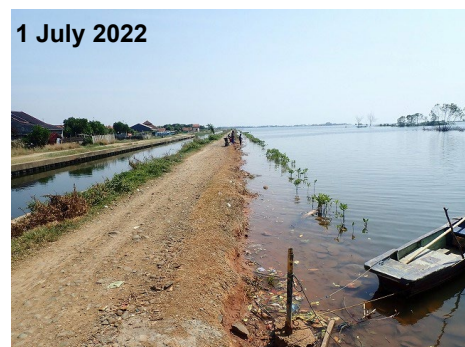
Protection Dike against Tidal Flood (Titik P2 gambar di atas)
