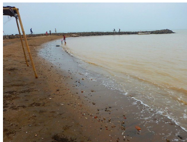
The shore behind the breakwater reached to the breakwater
