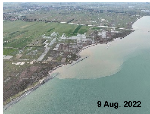
Silt Diffusion due to Land Erosion (P2)
