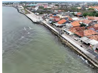
Coastal Protection at Urban Area (Line Protection)
