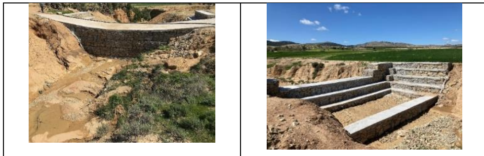
Figure 18-22 Case of Erosion Prevention Measures against Gully Erosion in Upstream of Siliana River
