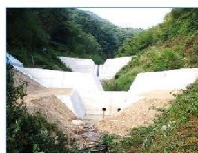
Series of check dam in the nearest valley
