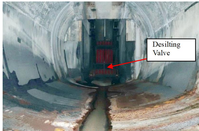
Figure 9-7 Visual inspection of the channel section of the existing sediment discharge facility (as of 2017)
