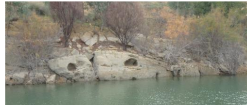
above : Partial erosion of sandstone below : Overall view
