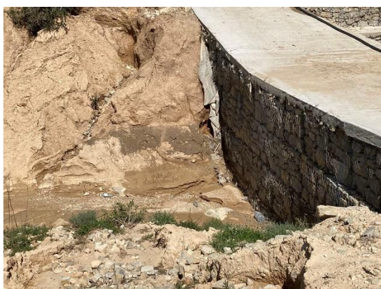
Check dam in the branch of Siliana river (2022.3)
