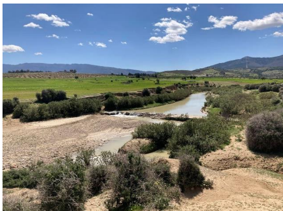
Siliana River (from downstream) (2022.3)
