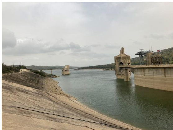
Zone A (Spillway) (2022.3)
