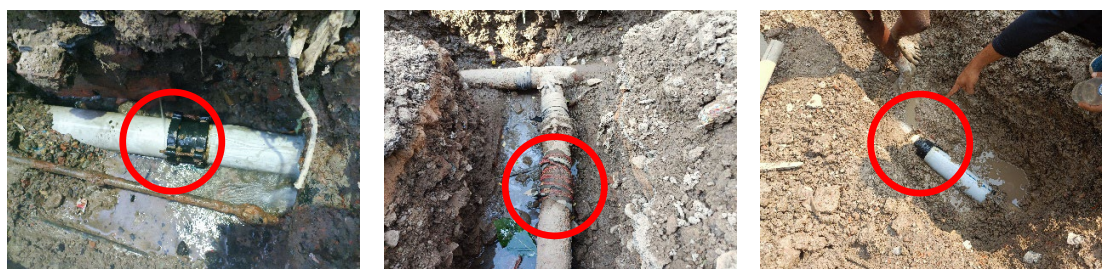
Figure 7-1. Leakage point
