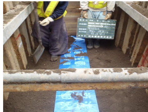
Figure 8-7. Pipe alert sheet
