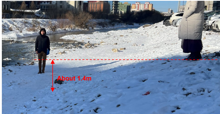
(Flooded Area in July 2023 Flood) Embankment height: approximately 1.5m
