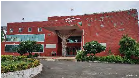
Appearance of TBGP Office Building in Chennai
