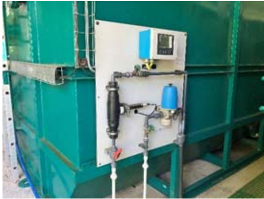
Figure 5-13 Water Quality Measuring Instruments and SCADA in Antrim WTP
