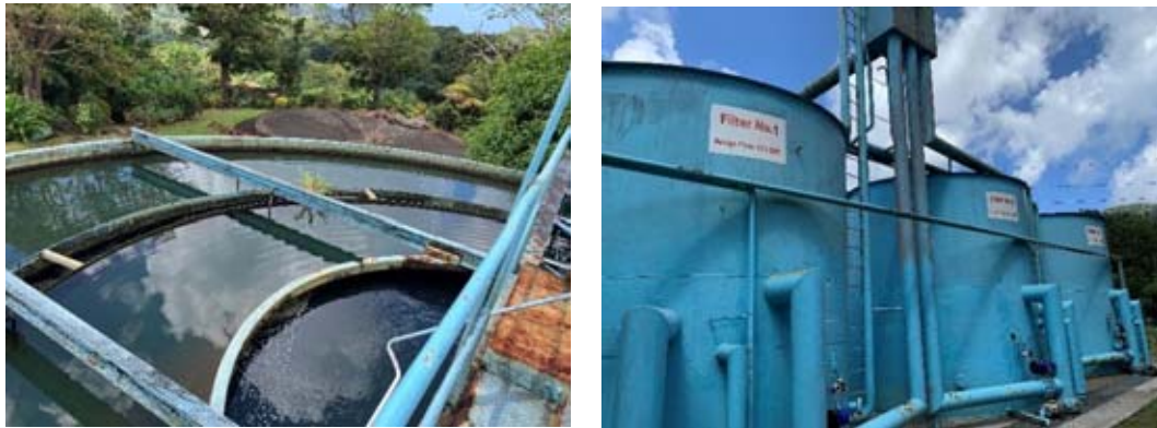
Figure 8-10 Annandale WTP (left: clarifier, right: rapid sand filter)
