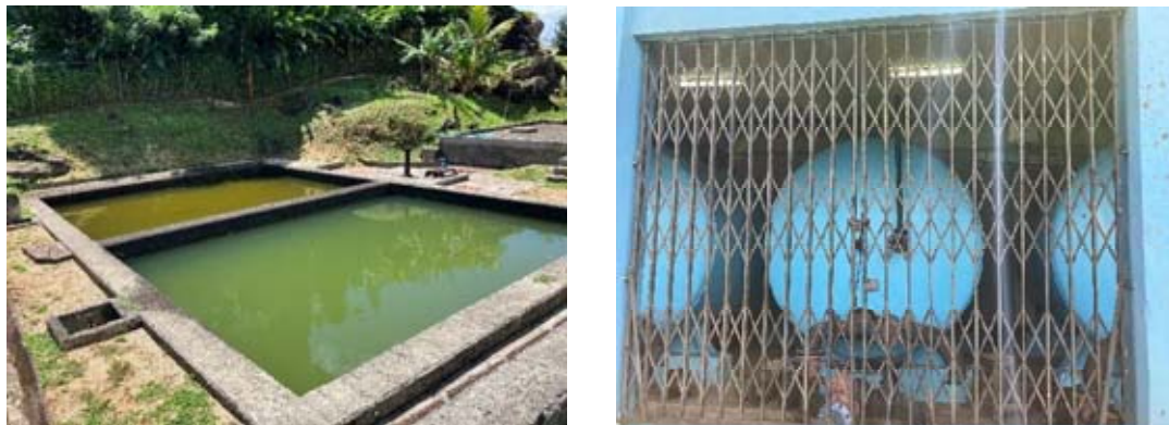
Figure 8-11 Vendomme WTP (left: slow sand filter, right: pressure filter)
