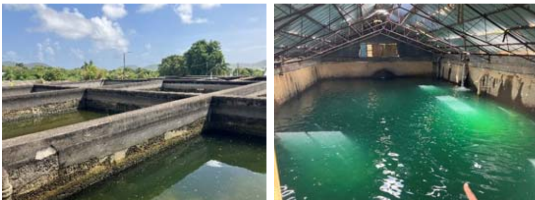
Figure 6-7 La Guerite WTP (left: sedimentation tank, right: clear water reservoir)
