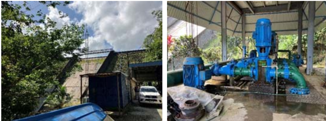
Figure 3-19 John Compton Dam and pump facilities for low water level
