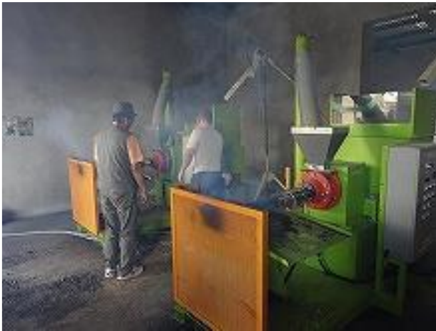
Grind Mills at the Mbeya project site. (Source: JICA)
