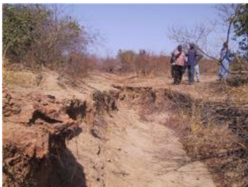
Water erosion (photo: JICA)
