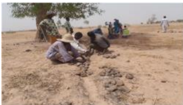
Construction of stone barriers (photo: JICA)
