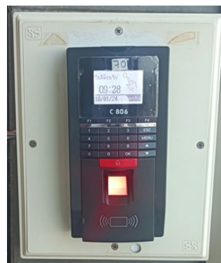
(b) NCC system server room
