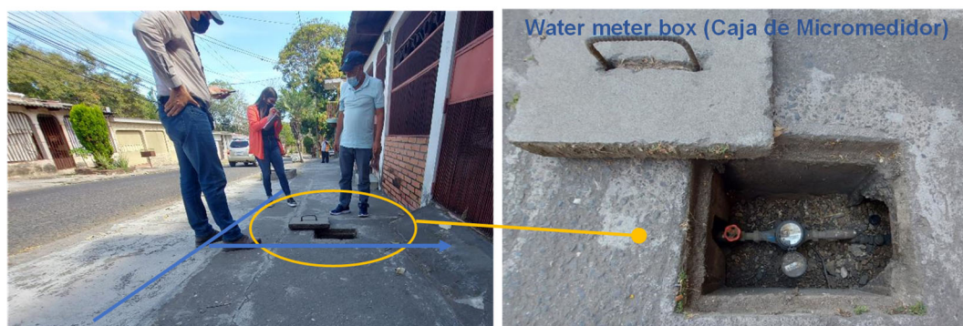
Figure 3.3.6 Installation of Water Meter
