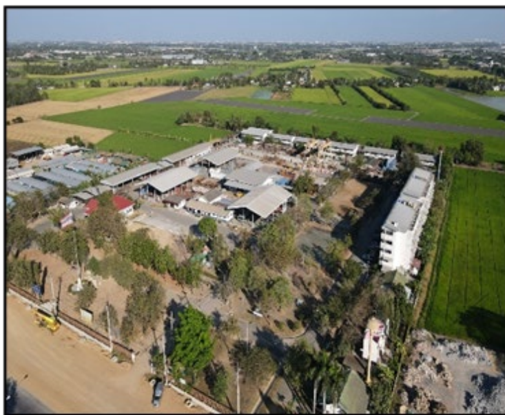
図 5.3 Bridge Construction and Rehabilitation Center3 (BCRC3) の全景 294
