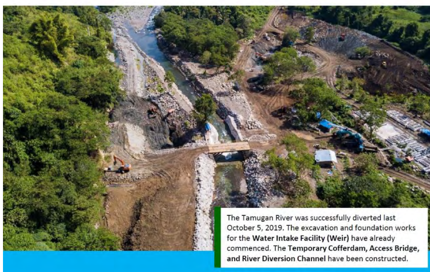
Figure 3.4.3-12 Construction of Intake Weir in Tamugan River
