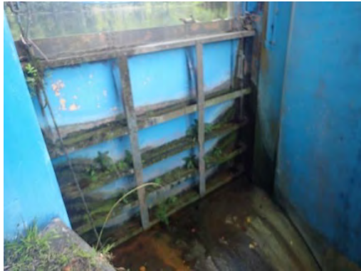
Spillway Gate in Buhisan Dam
