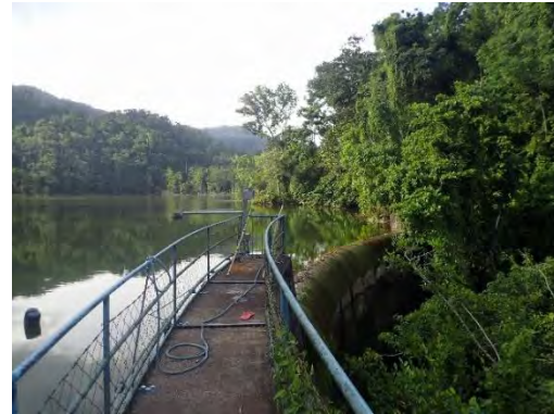
Ogee crest spillway in Buhisan Dam
