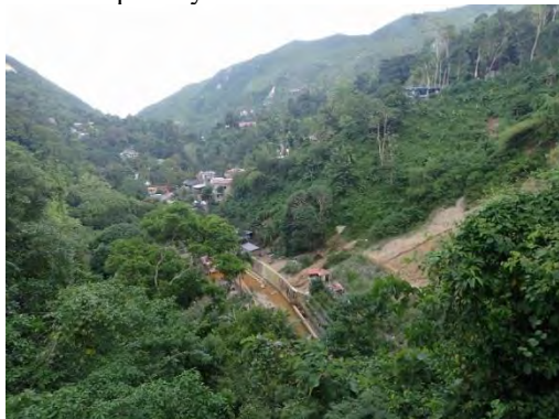
Downstream view of Buhisan Dam
