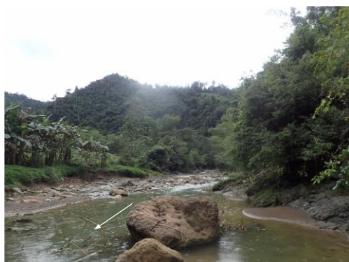
Site Inspection to Kotkot Dam Site Dec. 09, 2022
