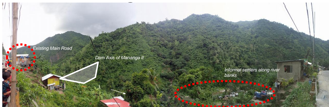
Site Inspection to Mananga II Dam Site Dec. 09, 2022
