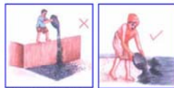
Concrete should not be thrown from height Concrete should be placed from little height
