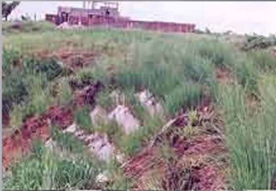
Stabilizing a cliff, Oaxaca, Mexico
