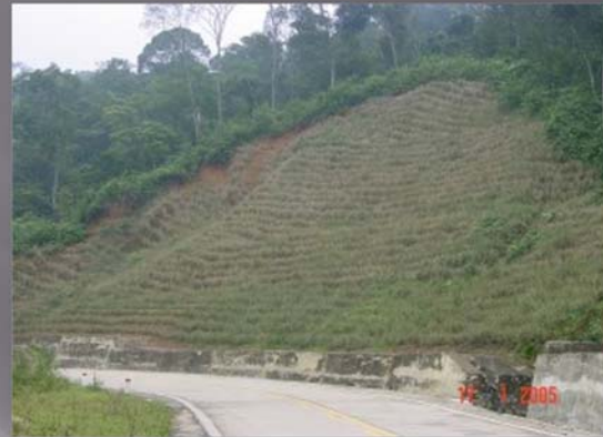
Extreme slope stabilization Ho Chi Minh Highway, Vietnam
