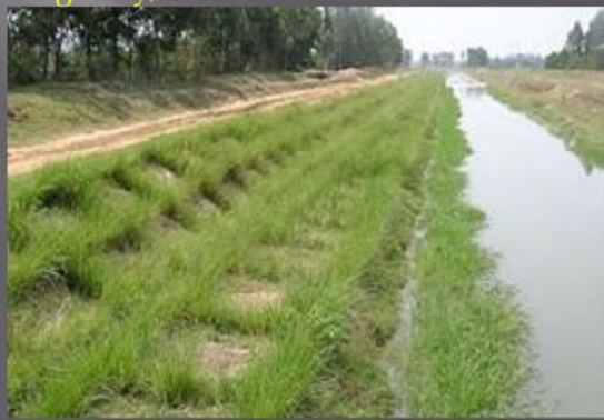
Canal bank stabilization, Central Vietnam
