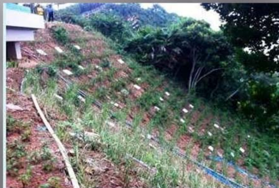
Soil nail with vetiver, Vietnam
