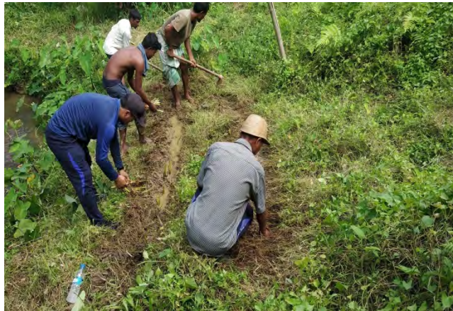
Demonstration of vetiver grass planting in the river bank for soil erosion control at stream bank.
