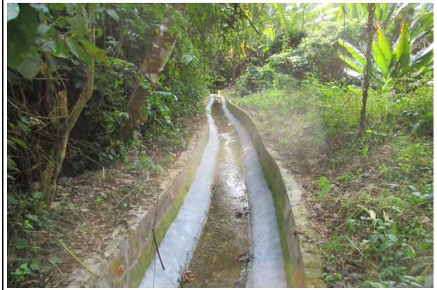
Construction of main channel haunch to prevent leakage from channel corner
