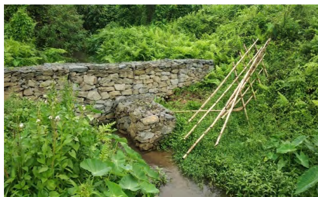
Construction of check Dam for soil erosion control at stream bank.
