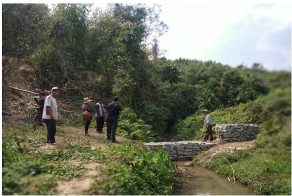
Supervision of check dam during the construction period.
