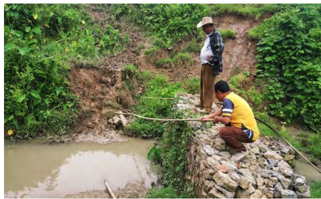
Checking the condition and effectiveness of check dam construction by the field officers from LRS&WCD
