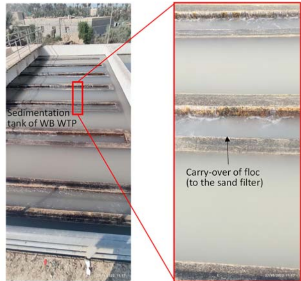
Figure 4.7 Sedimentation Tank of WB WTP
