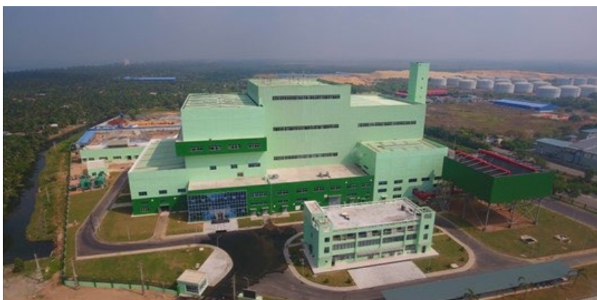
Figure 2-8 Western Power Kerawalapitiya (WPK) WtE facility
