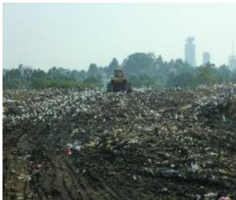
Kotikawathatha PS The disposal site is managed by the LA. The site is adjacent to the town area. Waste disposed at site is managed by pushing and pressing by bulldozer.
