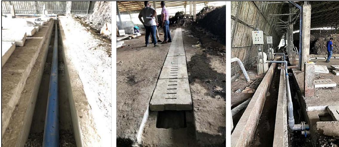
Figure 12 Construction of below ground forced aeration system
