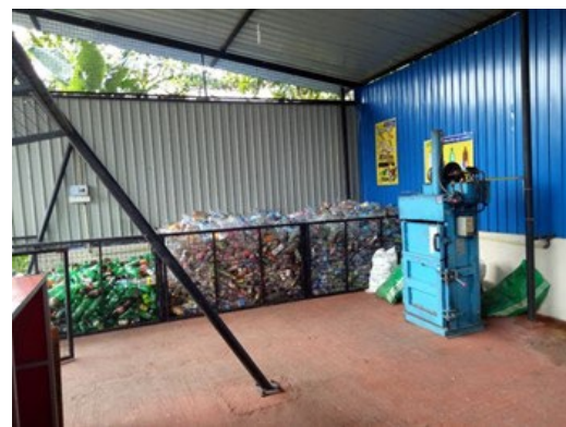
Recyclable sorting and storing center operated by Biyagama PS
