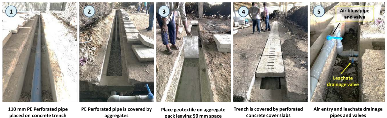
Figure 14 Laying of PE aeration pipe on the concrete ditch
