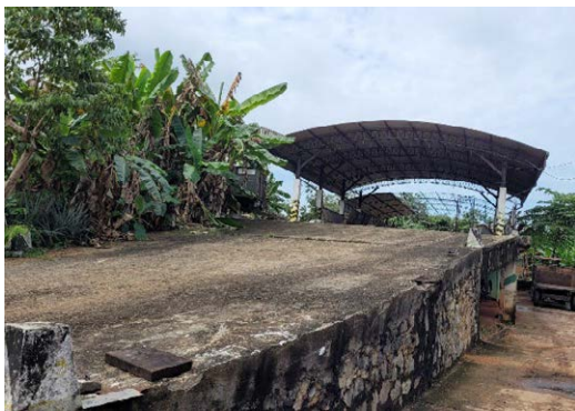
Transfer station entrance ramp
