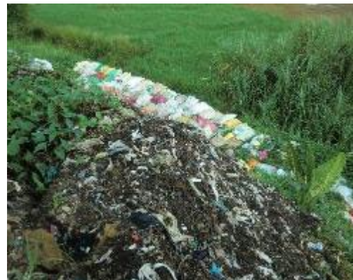
Agalawatta PS Residual materials remaining after sorting recyclables from other waste are packed in bags and used as earth retaining walls for disposal sites.
