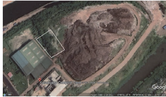
Composting plant and final disposal site (Site A)
