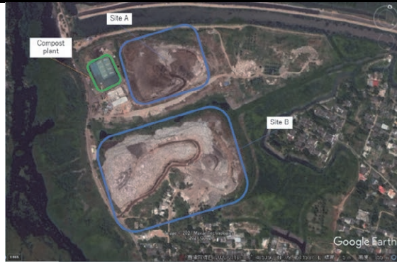
Karadiyana final disposal site
