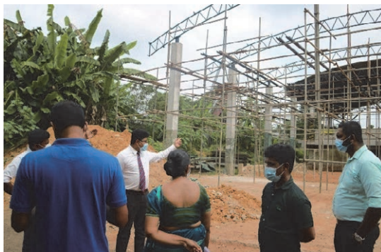
Monitoring at the transfer station under construction
