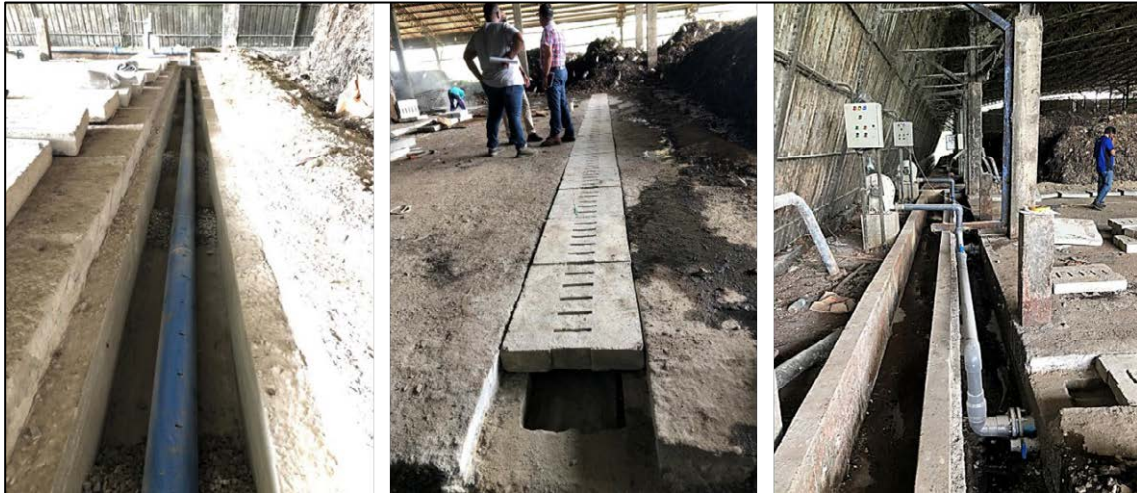
Figure 12 Construction of below ground forced aeration system
