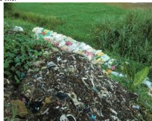
Agalawatta PS Residual materials remaining after sorting recyclables from other waste are packed in bags and used as earth retaining walls for disposal sites.
