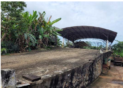
Transfer station entrance ramp
