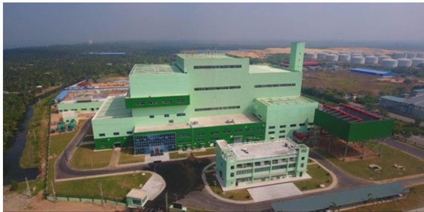
Figure 2-8 Western Power Kerawalapitiya (WPK) WtE facility
