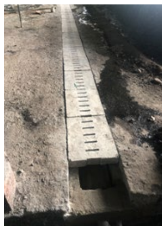
Perforated pipe laying in trench for below the ground aeration system
