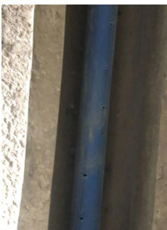
Perforated pipe laying in trench for below the ground aeration system
