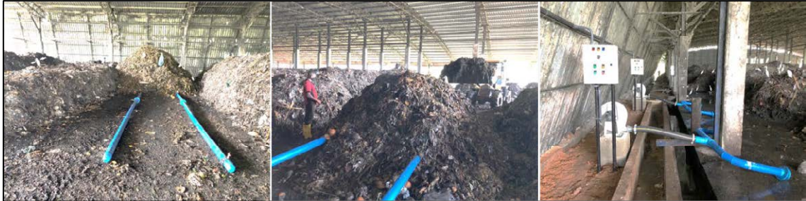
Figure 11 Construction of static piles for the above ground forced aerated pipes
