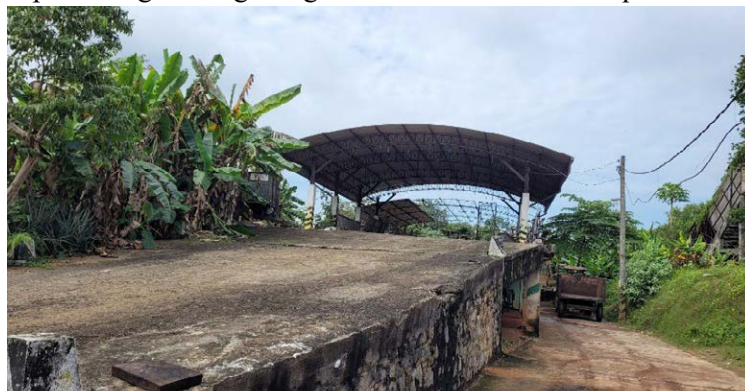
Figure 3 ramp and a roofed area for Kalutara Transfer Station
