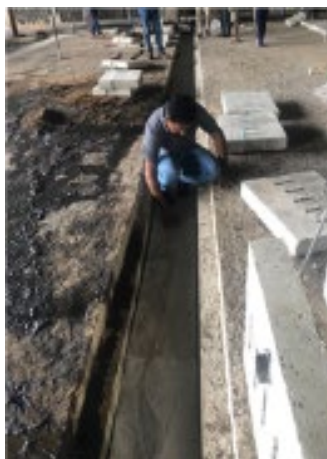
Perforated pipe laying in trench for below the ground aeration system
