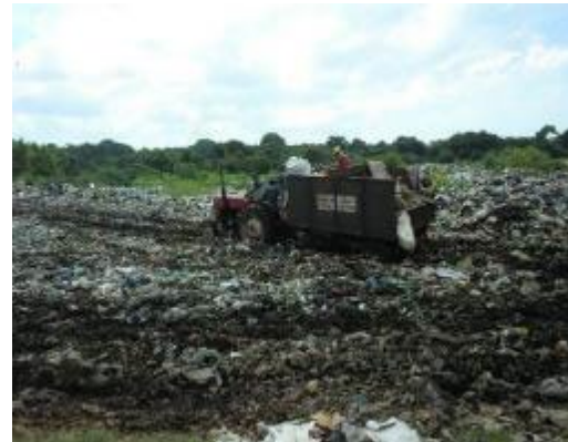
Katunayake Seeduwa UC The disposal site maintenance by heavy equipment twice a month. However, as access roads for collection vehicles are not properly maintained, only tractors are able to enter the site.
