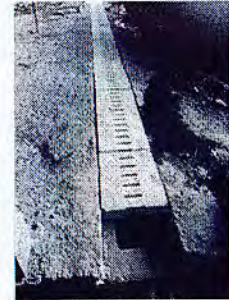
Laying the perforated PVC pipes in covered trenches
