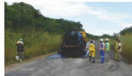
Photo: Road Maintenance by DOR
