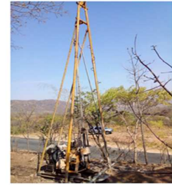
Photo: Boring survey
