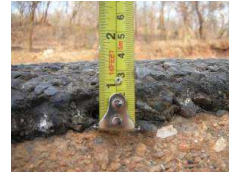
Photo: Existing pavement surface
