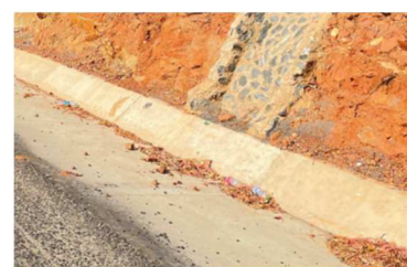
Photo: Phase 1 maintained ditches
