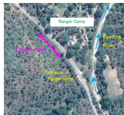
Photo: Existing road beside the river
