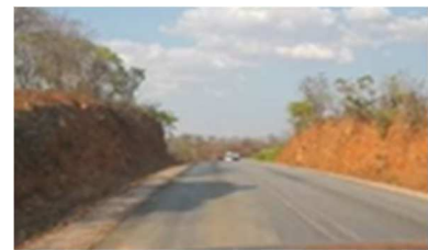
Photo: Difficult to put detour
