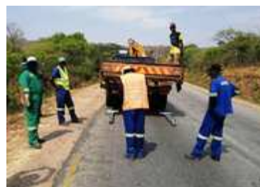
Photo: Benkelman beam survey
