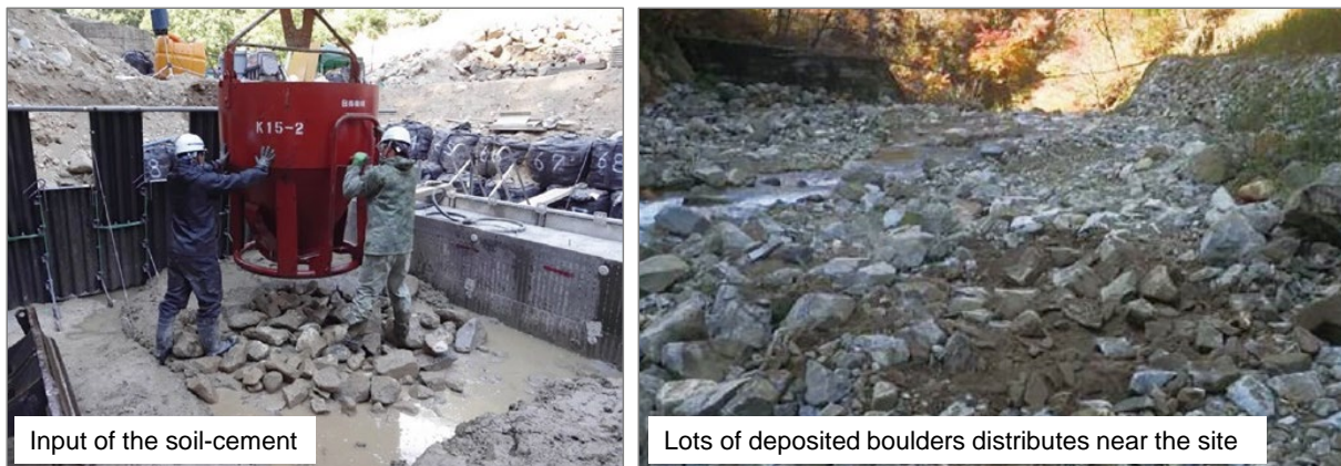
Figure 4.6.4 Example of Use of Soil-Cement Method in “Sabo” Dam Construction Site of Japan
