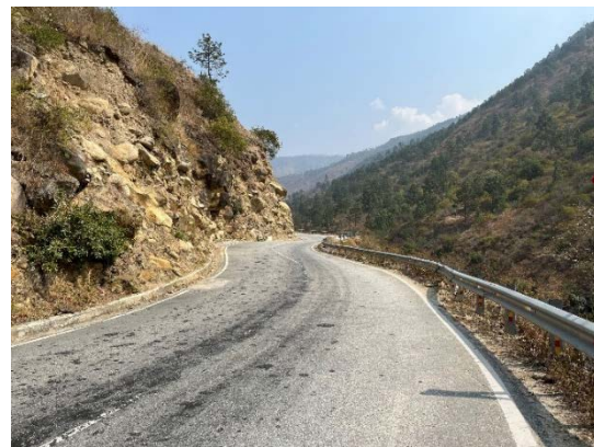
Road situation (Trashigang side)
