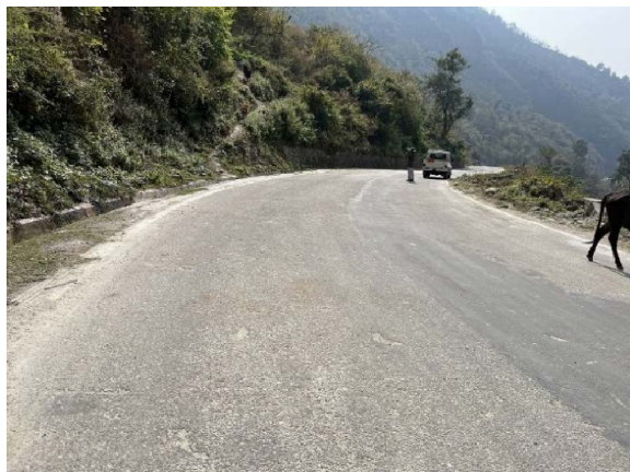
Road situation (Trashigang Side)
