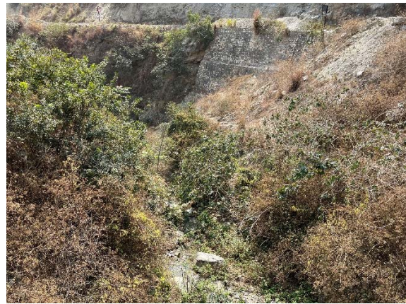
Downstream side of the existing bridge
