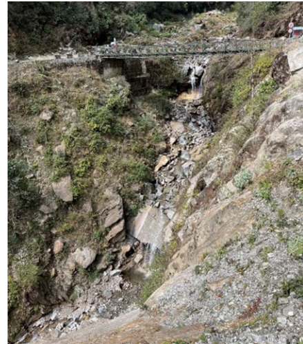
Downstream side of the existing bridg
