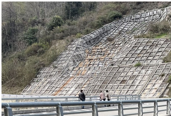
Slope protection (Teleganchu Bridge)
