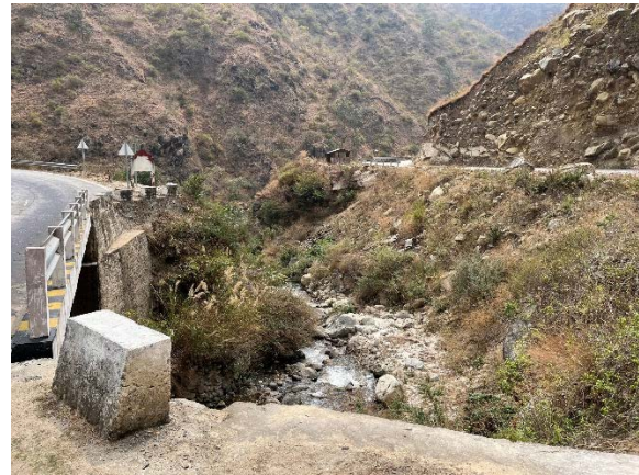
Downstream side of the existing bridge
