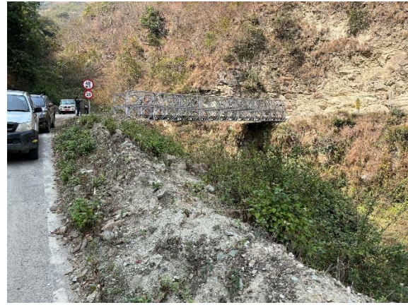
Downstream side of the existing bridge
