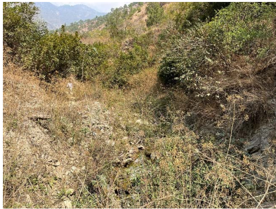
Upstream side of the existing bridge
