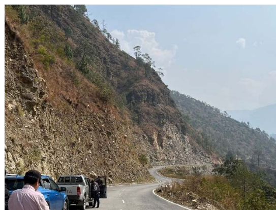
Road situation (Trashigang side )
