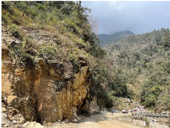
Right slope (Trongsa side)
