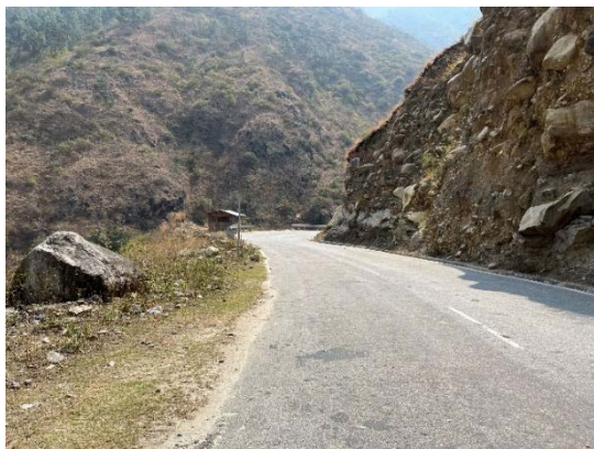
Road situation (Mongar side)
