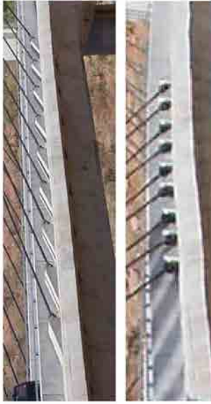
Fig. 7 Photographs of Anchorages (on Girder)
