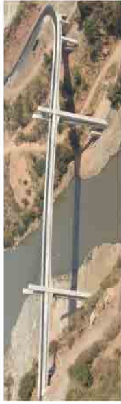
Fig. 1 General View and Overview Photo of the New Abay Bridge
